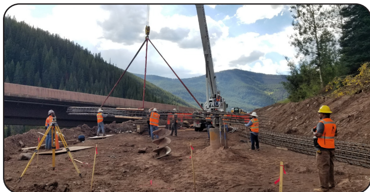
Image 23 & 24. Drilled Shafts and Setting Rebar Cage Abutments for Pier 2 at I-70 WB over Polk Creek (F-12-AT)
