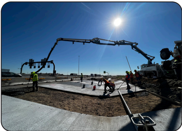
Image 17. Construction on Central Park Blvd.
