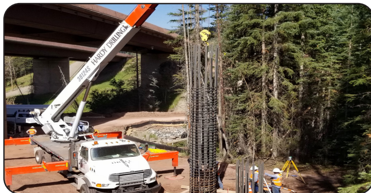
Image 23 & 24. Drilled Shafts and Setting Rebar Cage Abutments for Pier 2 at I-70 WB over Polk Creek (F-12-AT)
