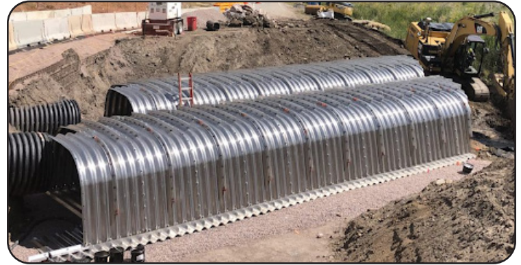
Image 19 & 20. Installation of an Aluminum Box Culvert at US 9 over Mack Gulch (J-15-G)
