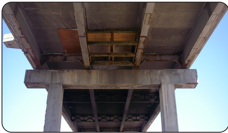
Image 7 & 8. Full-depth Deck Repairs to I-25 ML SB over US 160 ML, RR Spur (N-17-AD)
