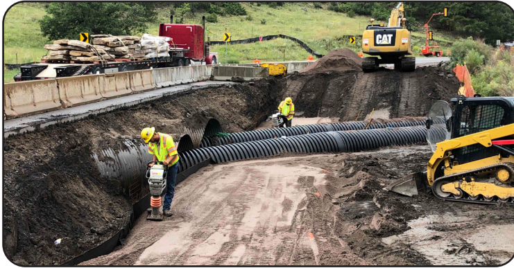
Image 19 & 20. Installation of an Aluminum Box Culvert at US 9 over Mack Gulch (J-15-G)
