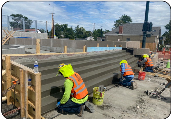
Image 16. Construction on the Cover Top
