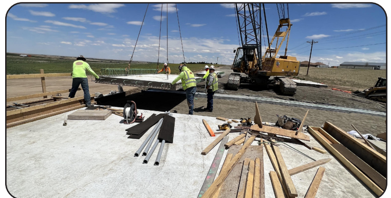
Image 21 & 22. Bridge Deck Rebar and Pre-cast Bridge Approach Installation on US 36 ML over Draw (F-19-E)
