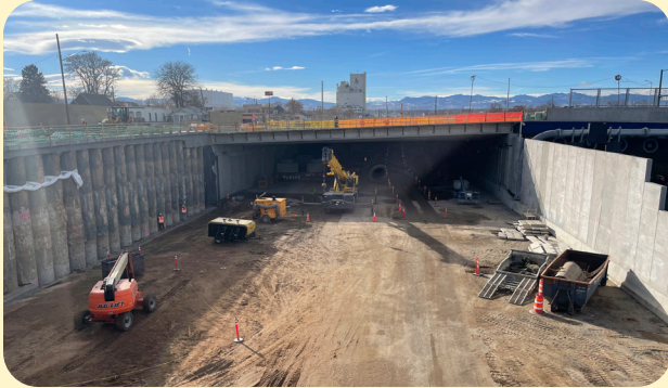
Image 14. Eastbound I-70 Future Lowered Lanes
