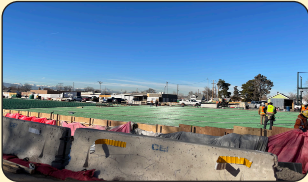
Image 13. Deck rebar for the Eastbound I-70 Lanes Cover
