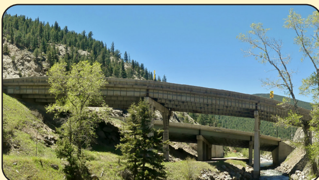
Image 18. I-70 over US 6 and Clear Creek in Clear Creek County (F-15-BL)
