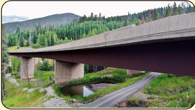
Image 19. I-70 EB over Polk Creek in Eagle County (F-12-AS)
