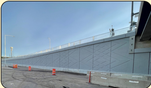
Image 15. Eastbound I-70 Onramp at 46th Ave.
