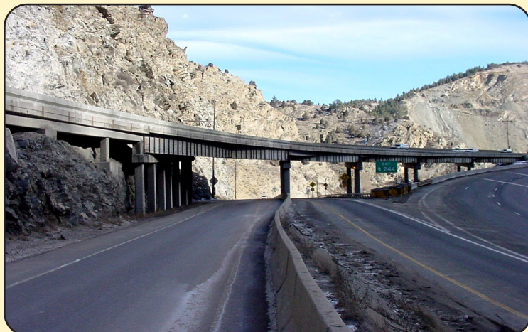
Image 3. I-70 ML over US 6, Clear Creek in Clear Creek County (F-15-BL)
