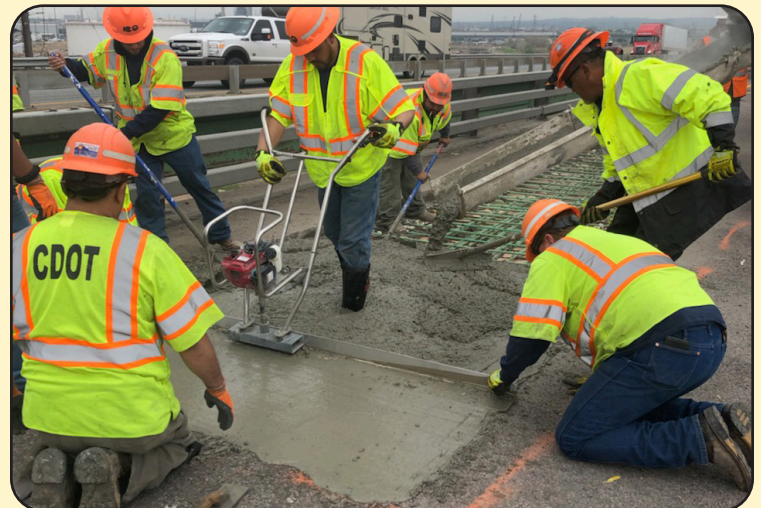
Image 6. Emergency Repairs to I-270 ML WBND over SH 265 ML & UPRR (E-17-IH)
