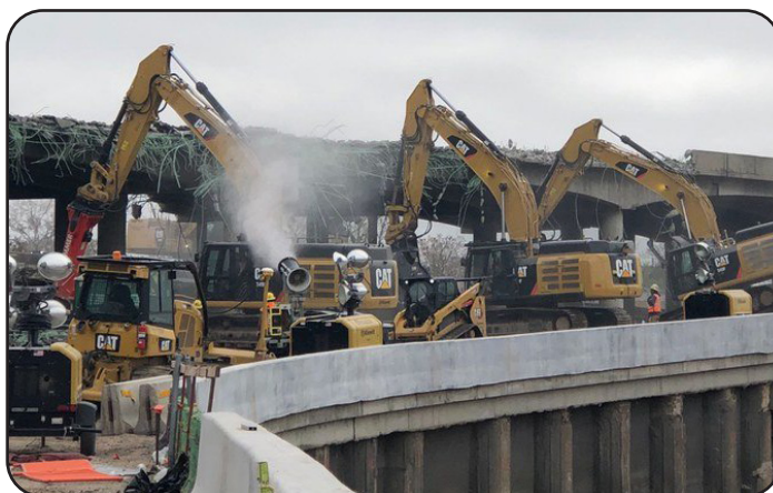
Image 4. Demolition of the I-70 Viaduct
