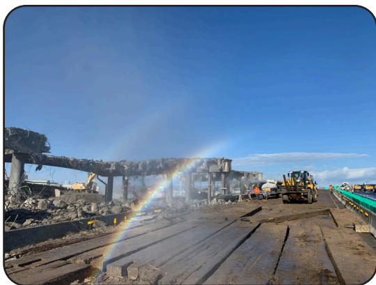
Image 20. Demolition of the I-70 Viaduct
