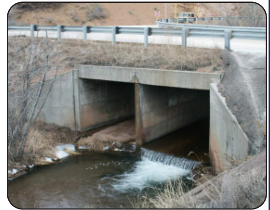
Image 21. US 24 Service Rd over Fountain Creek in El Paso County (I-17-X)
