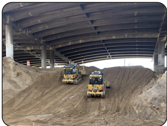
Image 18. Excavation of the Future I-70 East Bound Lanes
