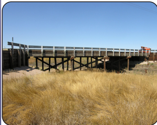
Image 22. SH 61 over Surveyor Creek in Washington County (D-25-E)
