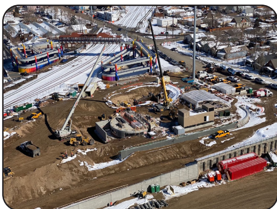
Image 16. Aerial of Pump Station near York Street
