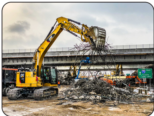
Image 14. Demolition of I-70 over Quebec Street Bridge
