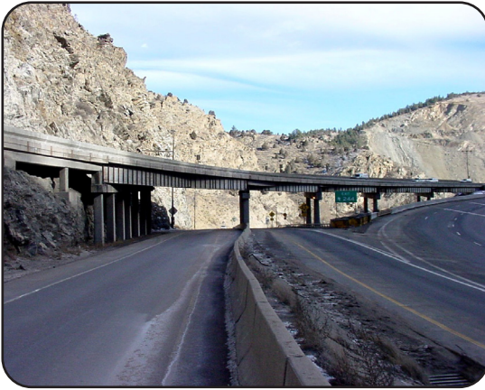
Image 20. I-70 over US6 and Clear Creek in Clear Creek County (F-15-BL)
