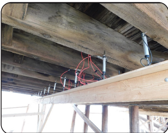
Image 22. Load Testing Sensors Measuring Displacement on US 36 over Vega Creek in Washington County
