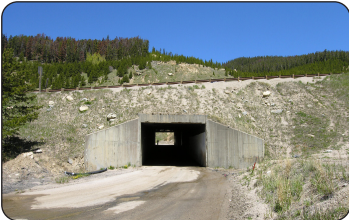
Image 7. I-70 over Forest Service Rd (F-13-S_Minor)
