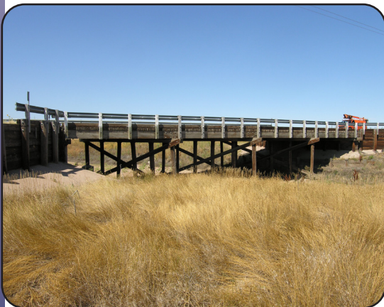
Image 18. SH 61 over Surveyor Creek in Washington County (D-25-E)
