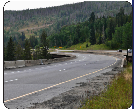
Image 21. I-70 over Polk Creek in Eagle County (F-12-AS)
