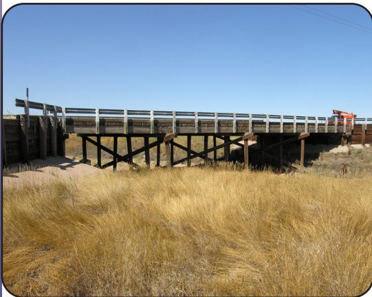
Image 17. SH 61 over Surveyor Creek in Washington County (D-25-E)
