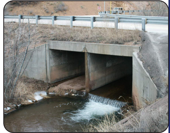
Image 16. US 24 Service Rd over Fountain Creek in El Paso County (I-17-X)
