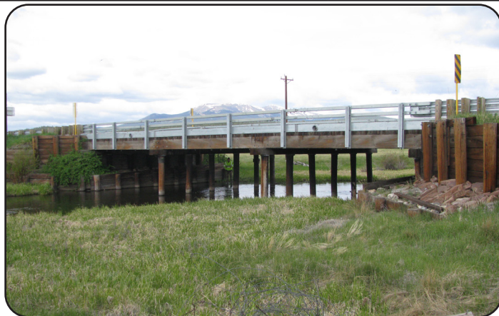
Image 2. US 285 over S. Fork S. Platte River in Park County (H-13-G)
