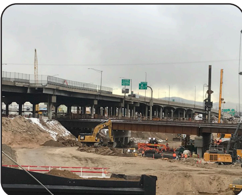
Image 15. Excavation at the York Street and UPRR Structures
