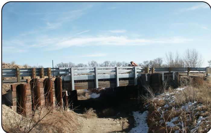
Image 4. SH 71 over Highline Canal in Otero County (M-22-N)
