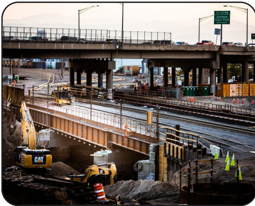
Image 13. Construction of the UPRR Bridge over I-70
