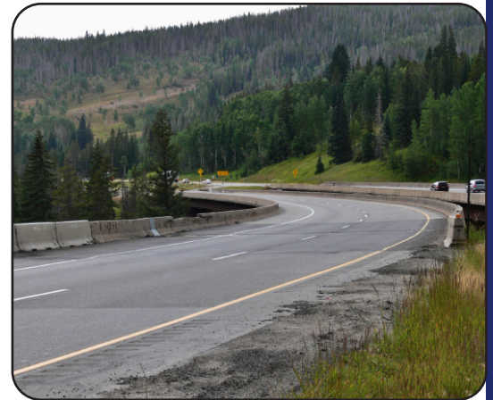
Image 20. I-70 over Polk Creek in Eagle County (F-12-AS)
