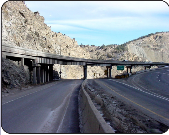
Image 19. I-70 over US6 and Clear Creek in Clear Creek County (F-15-BL)
