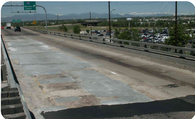
Image 1. Concrete Patch Deck Repairs on I-76 over York St
