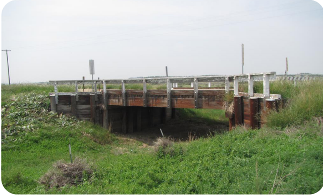
Image 5. SH 101 over Draw in Bent County Viewed from the West (M-24-A)
