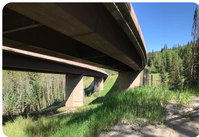
Image 6. I-70 EB over Polk Creek in Eagle County
