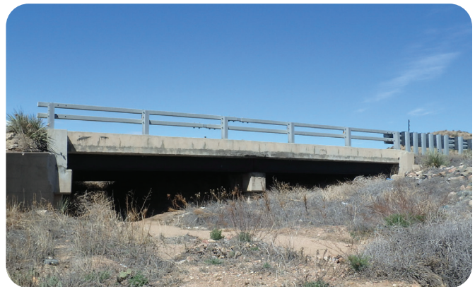
Image 2. US 34 over N Fork Republican River in Yuma County
