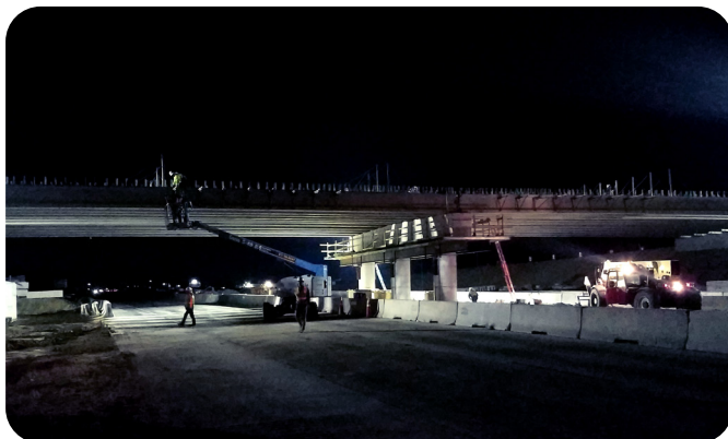
Image 3. Construction of County Road 48 over I-25
