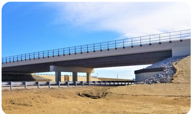
Image 4. Completed County Road 48 over I-25
