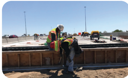
Image 10. Preparation and Pavement of the I-270 Flyover Bridge
