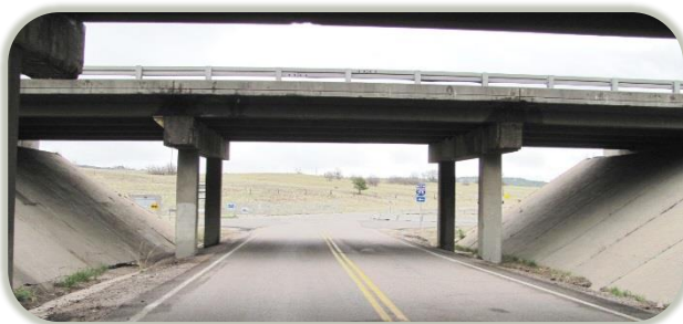
Image 1. Existing I-25 NB over County Rd (H-17-CH)
