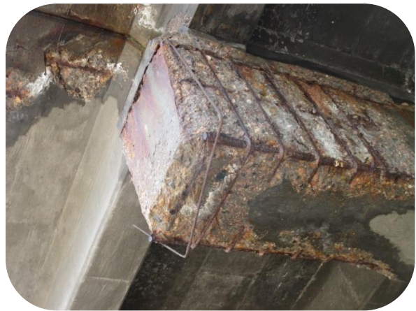
Image 6. H-17-CI Pier Cap Deterioration
