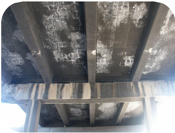
Image 5. H-17-CI Typical Deck Underside
