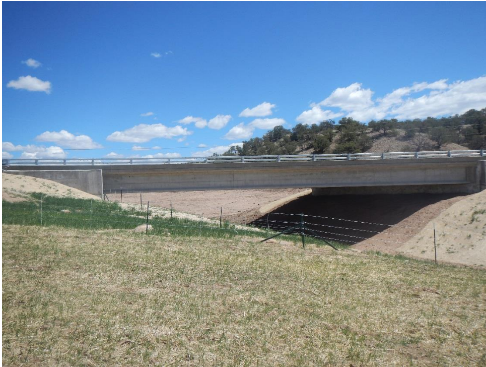
Image 3. SH 69 over Milligan Arroyo (M-16-P) Replacement
