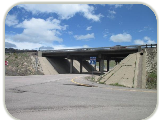
Image 2. Existing I-25 SB over County Rd (H-17-CI)
