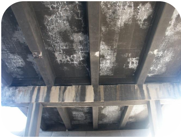
Image 7. H-17-CI Typical Deck Underside
