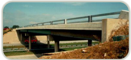
Image 4. Existing County Road 48 over I-25 (B-16-EU)
