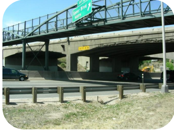
Image 10: South Elevation View of Speer Blvd Southbound over I-25 (E-16-EO)
