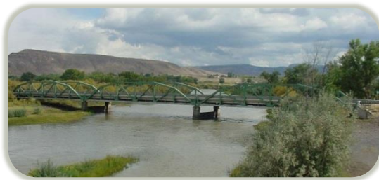
Image 1. Existing SH 92 over Gunnison River (I-05-V)
