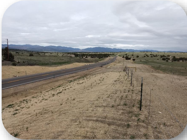
Image 5. SH 96 over Rush Creek (K-17-F) Replacement
