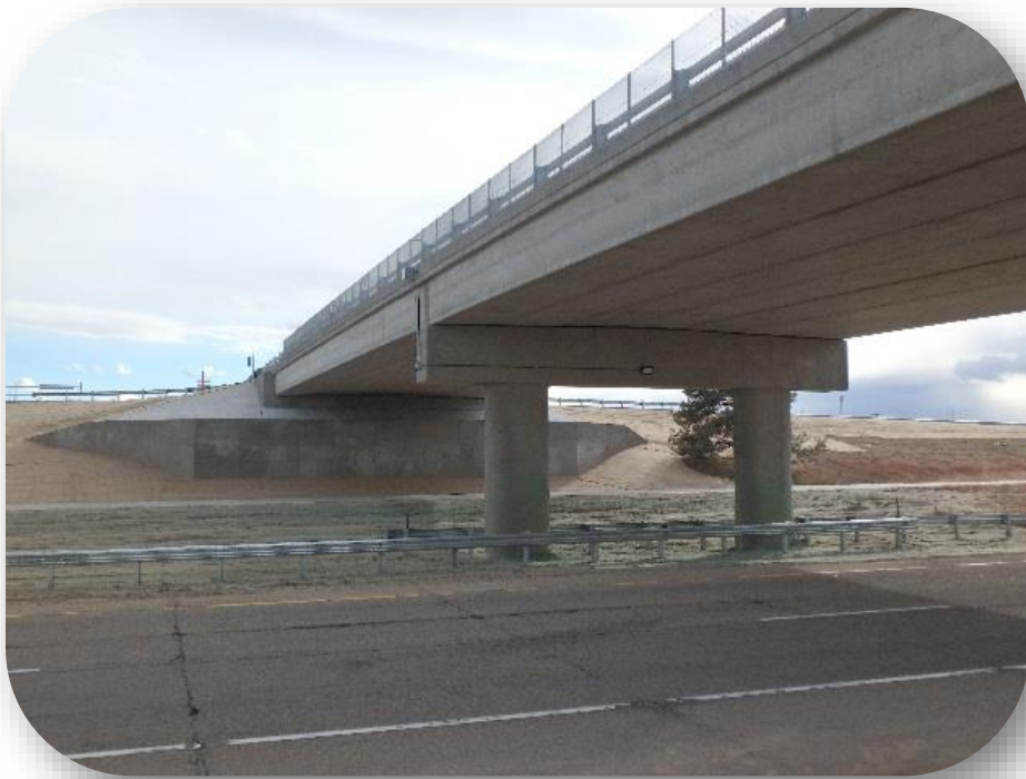
Image 5. US 59 over I-70 (G-25-K) Replacement
