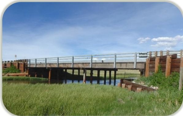
Image 2. Existing US 285 over South Fork South Platte River (H-13-G)
