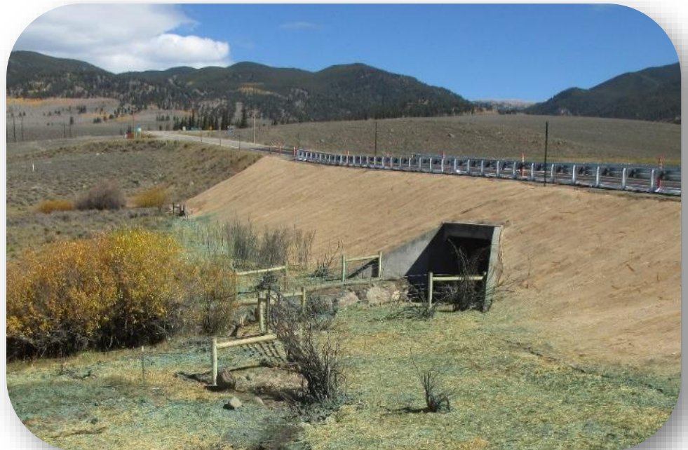
Image 6. US 50 over Agate Creek (K-11-G) Replacement
