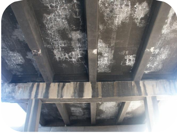
Image 8. H-17-CI Typical Deck Underside
