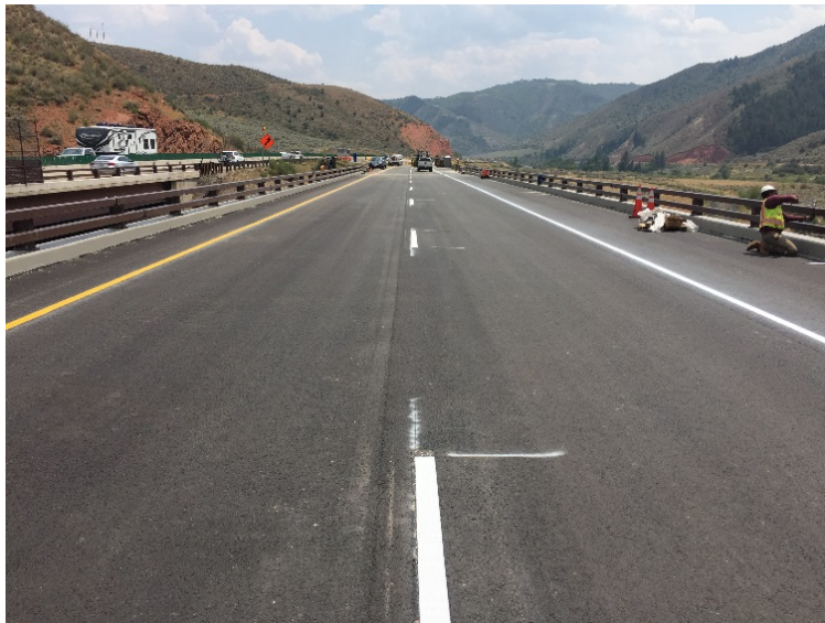
Image 5. F-10-L Rehabilitated Deck
