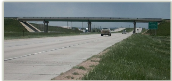
Image 2. Existing I-25 over County Road 48 (B-16-EU)
