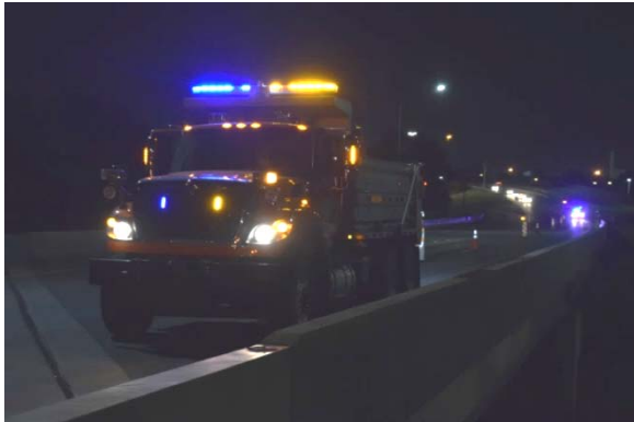
Photo 2. Load Testing of E-16-LU using Fully Loaded Dump Trucks
