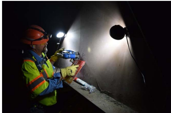
Photo 3. Installation of an Arrest Hole to Mitigate Fatigue Cracking
