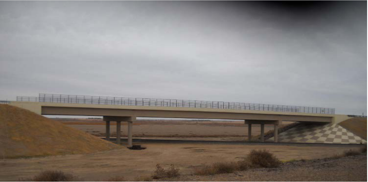
L-27-S and L-28-C, a $8.5M project, was completed in July.
