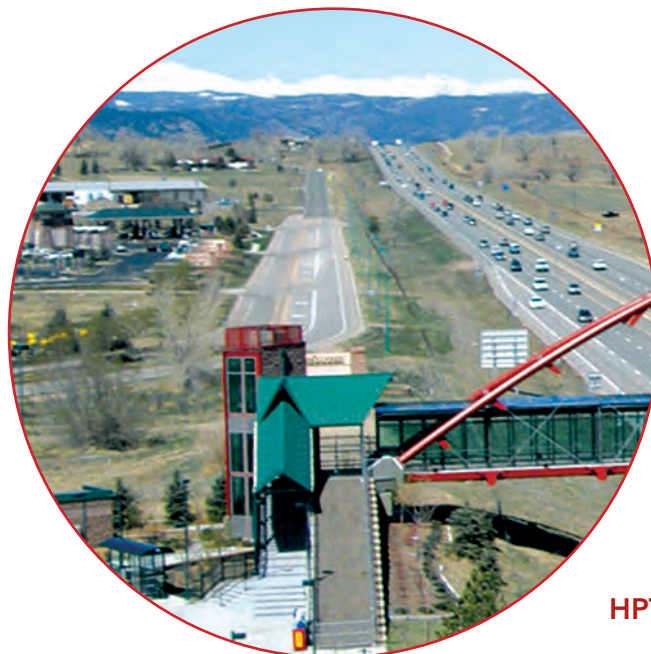
A view of US 36 looking west.
