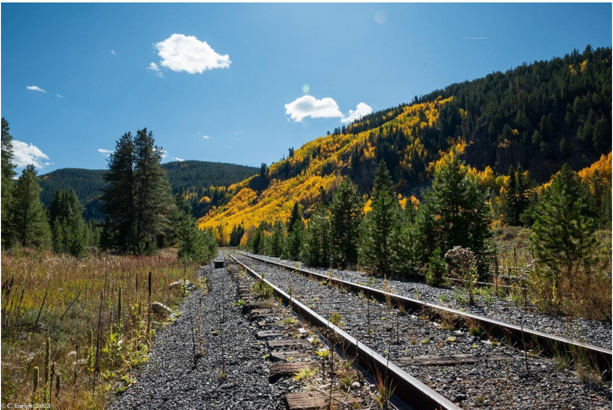
Figure 1: Tennessee Pass Subdivision at Camp Hale National Monument (C. Enright/CDOT)
