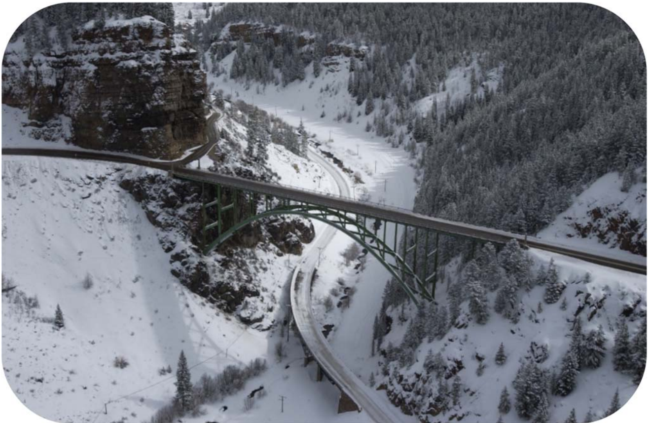
The Red Cliff Bridge in Eagle County, as seen in 2004, is Colorado’s only cantilevered steel arch bridge and is listed on the National Register of Historic Places.
