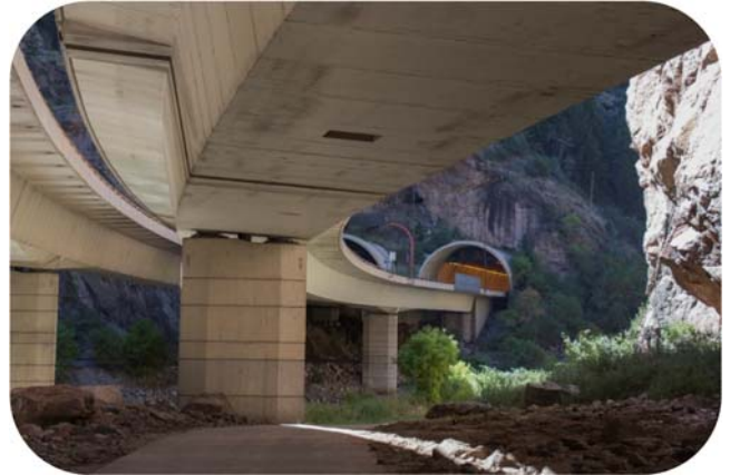
The Hanging Lakes Tunnel in Glenwood Canyon along Interstate 70. This stretch of Interstate completed the originally planned Interstate Highway System.
