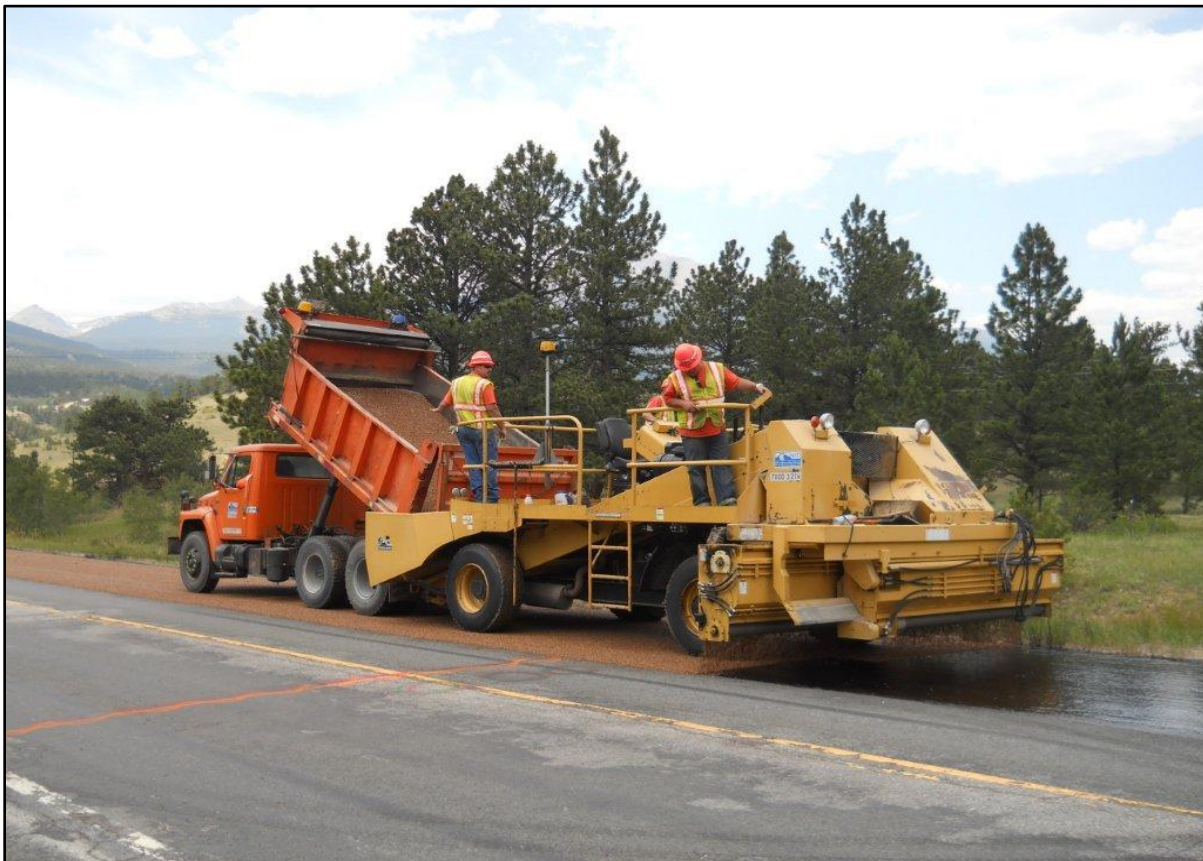
CDOT crew makes improvements to State Highway 7.
