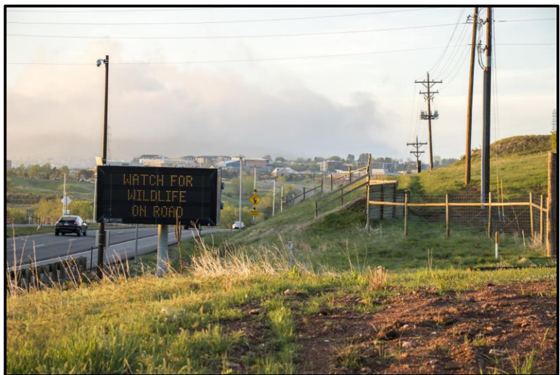
Investing in Variable Messaging Signs and other technologies is another strategy CDOT is using to prevent accidents and empower highway users to make more efficient travel decisions.
