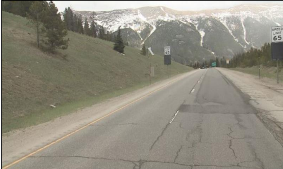
Interstate 70 near Copper Mountain. This stretch of pavement was last rehabilitated in 2009 and has a Drivability Life of one year.
