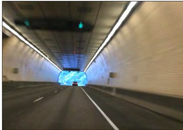
CDOT manages 21 tunnels statewide. Maintenance activities include washing the structures, ensuring electrical and ventilation systems are operating properly, and more.
