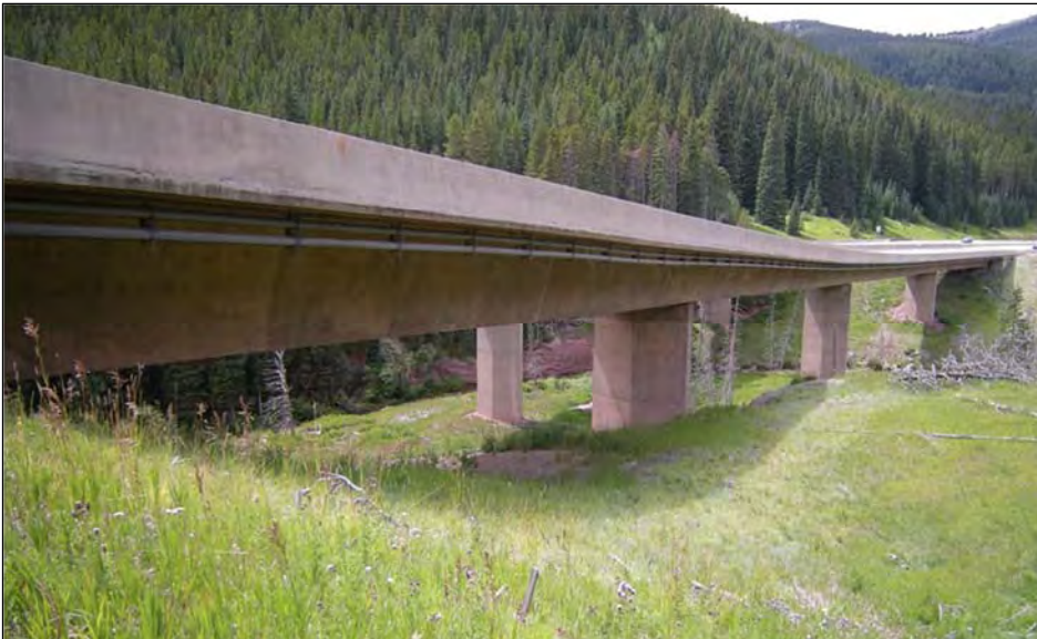
A bridge on Interstate 70 over Black Gore Creek near Vail.
