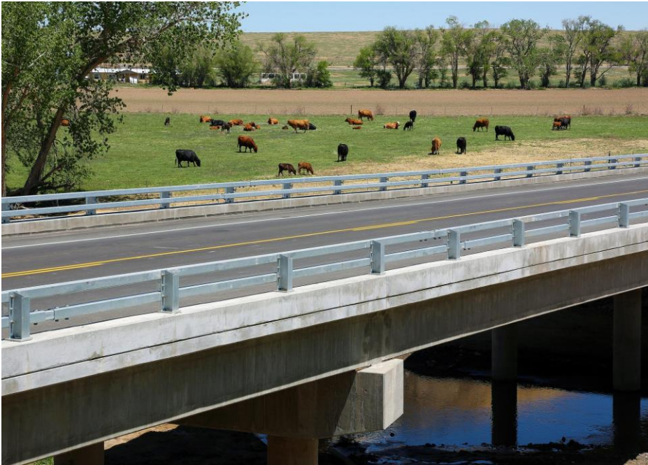
Bridge over the Purgatoire River in southern Colorado.
