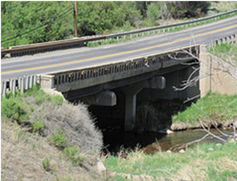
U.S. 6 Brush Creek Bridge
