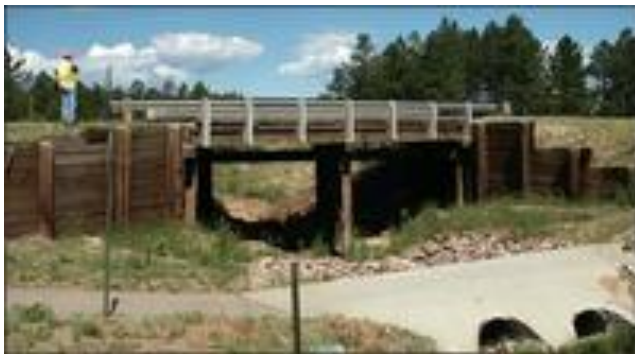
Loy Gulch Bridge
