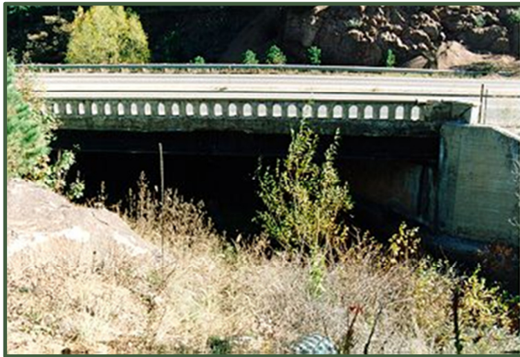
Fountain Creek Bridge
