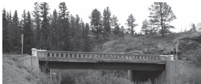
Twin Creek Bridge
