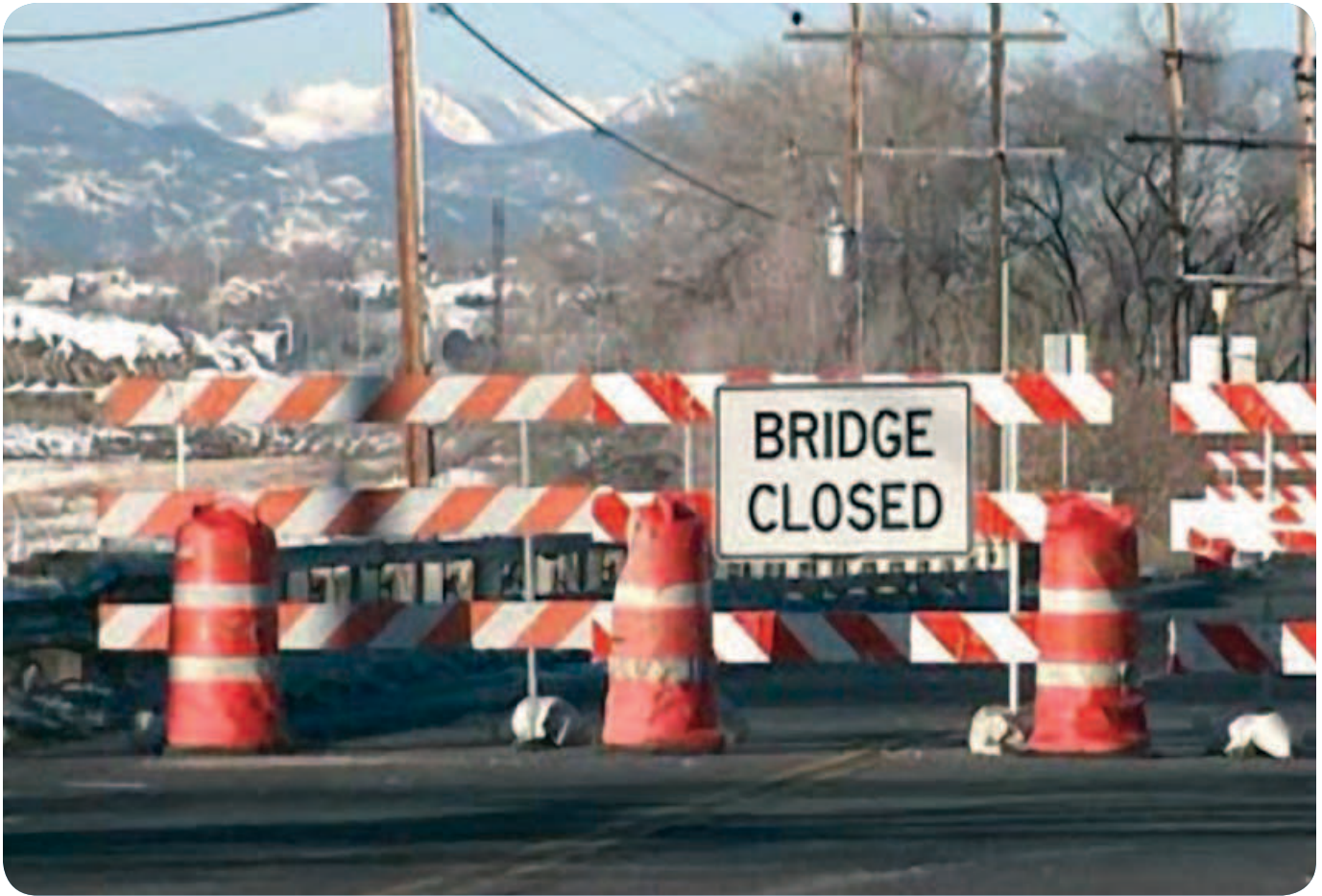
104 th Avenue Bridge over South Platte River
