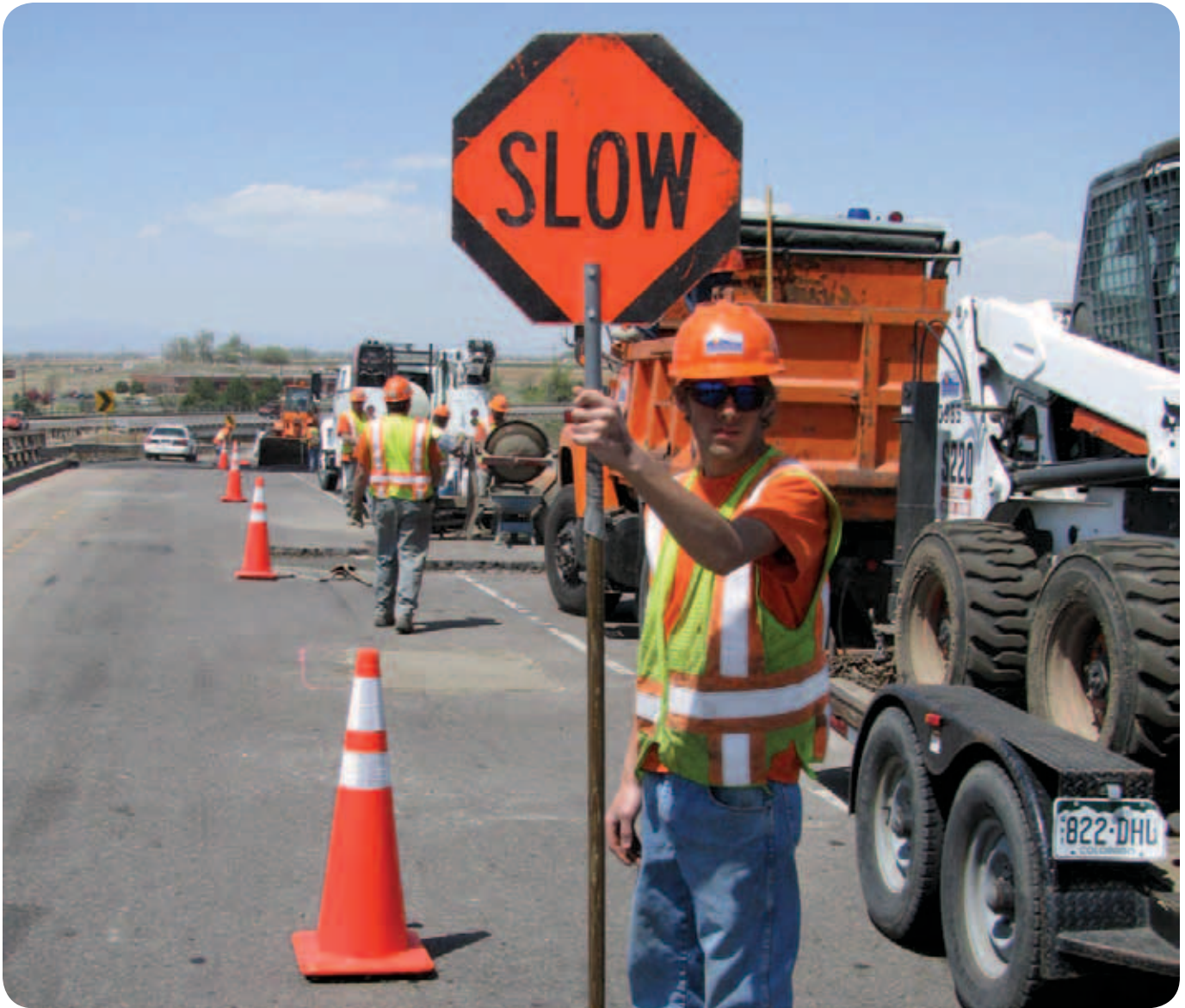
4 th Street bridge construction in Pueblo
