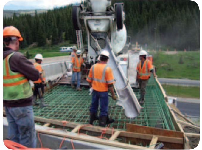
I-70 Shrine Pass Bridge
