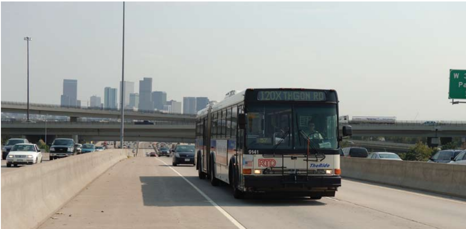
The I-25 Northbound Express Lane provides reliable travel times for buses, car pools and single drivers willing to pay a toll.
