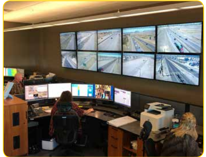
CDOT's new Regional Operations Center in Pueblo.
