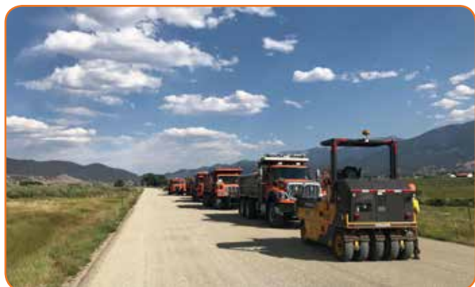
CDOT maintenance crews resurface CO 291 north of Salida.
