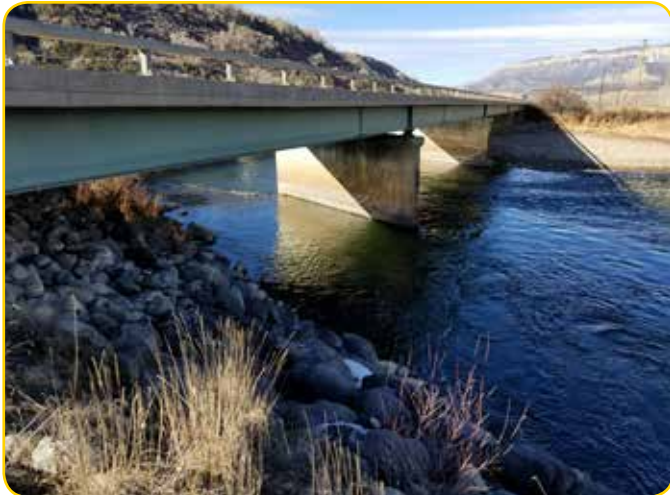
I-70 Colorado River Bridge at Rifle
