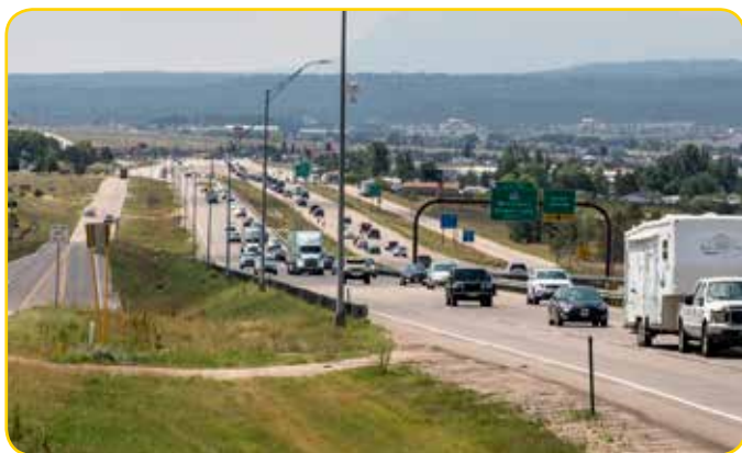
The I-25 South Gap project received contributions and support from El Paso and Douglas counties, as well as the Pikes Peak Rural Transportation Authority.
