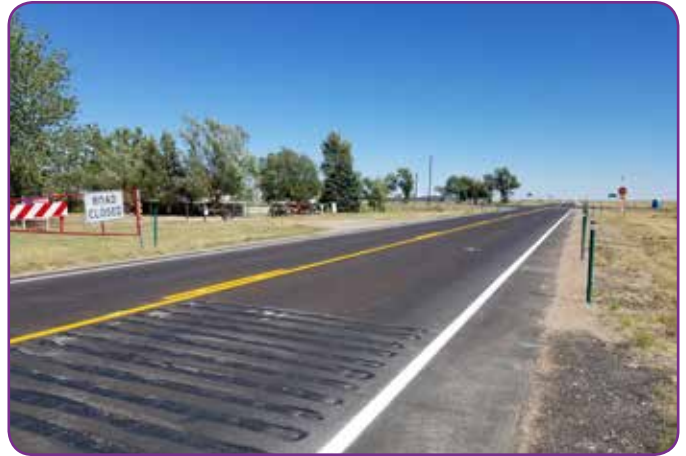
CO 71 at CO 90 in Punkin Center received safety upgrade.
