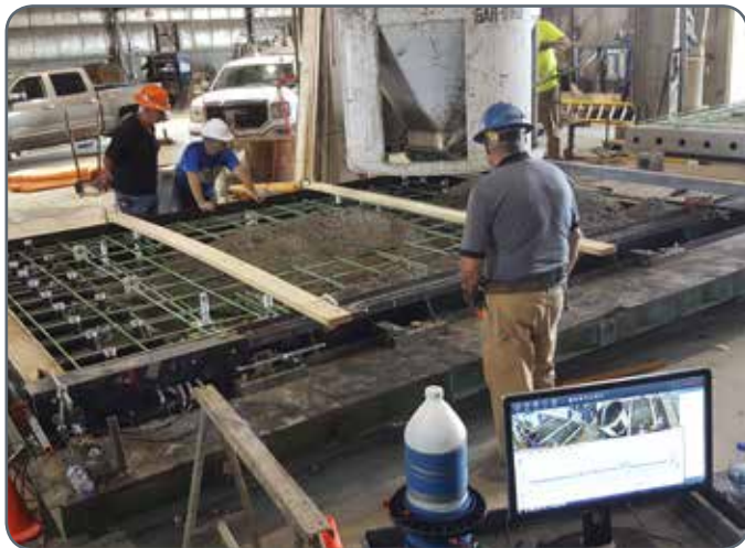
Smart pavement panels being fabricated.
