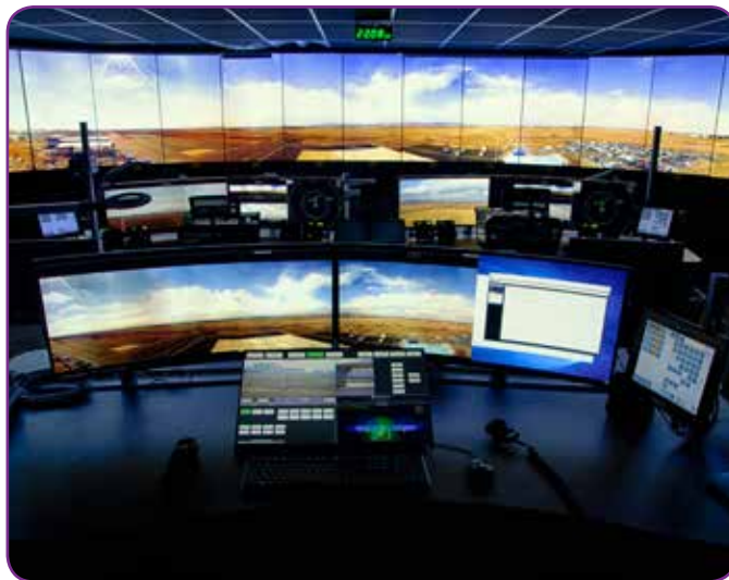
Remote Air Traffic Control Room at the Northern Colorado Regional Airport.
