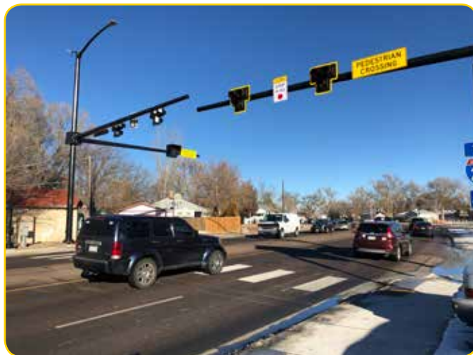
A modified High Intensity Activated Crosswalk (HAWK) beacon increases pedestrian safety at the intersection of Lincoln Street (CO 96) and Belmont Ave in Pueblo County.
