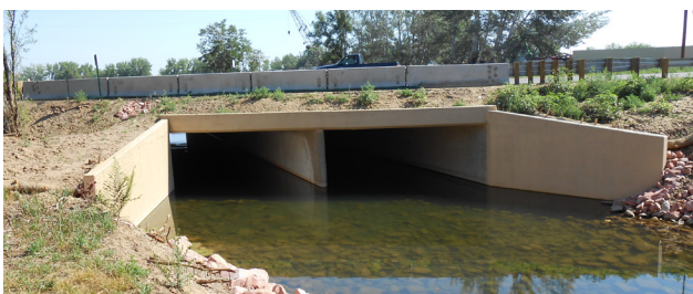
Dry Creek Bridge on US 287 in Ft. Collins was replaced with a concrete box culvert to meet new safety standards. [REGION 4]
