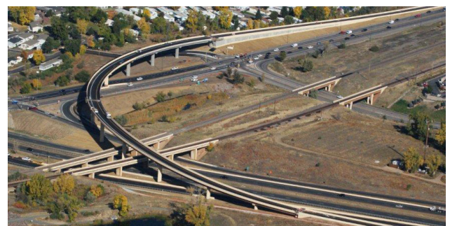
The new flyover from southbound Santa Fe Drive to eastbound C-470 provides a smoother connection at this heavily used interchange. In addition, a new climbing lane was constructed on eastbound C-470 to give motorists more time to reach travel speeds before merging with traffic. [REGION 6]
