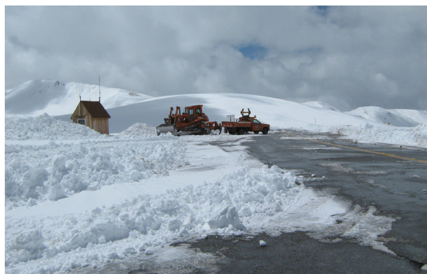
Crews worked around the clock to clear a late storm so SH 82 over Independence Pass could open by Memorial Day. [REGION 3]
