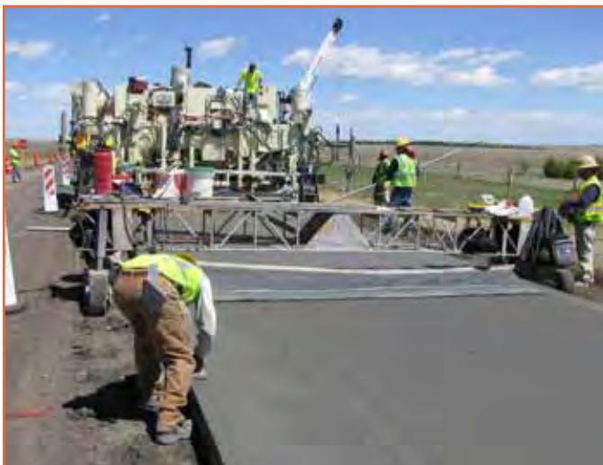
On US 385 in Yuma County, this project consisted of 8.5 miles of full-depth reclamation (removing the asphalt roadway down to a dirt surface), repaving with four inches of new asphalt, replacing 8.5 miles of fence and replacing two timber bridges with large concrete box structures [Region 4].
