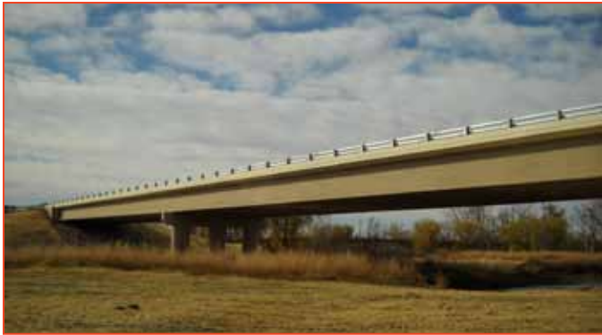
SH 89 Arkansas River Bridge, south of Holly, was replaced with $5.5 million in funding from the Colorado Bridge Enterprise [Region 2].
