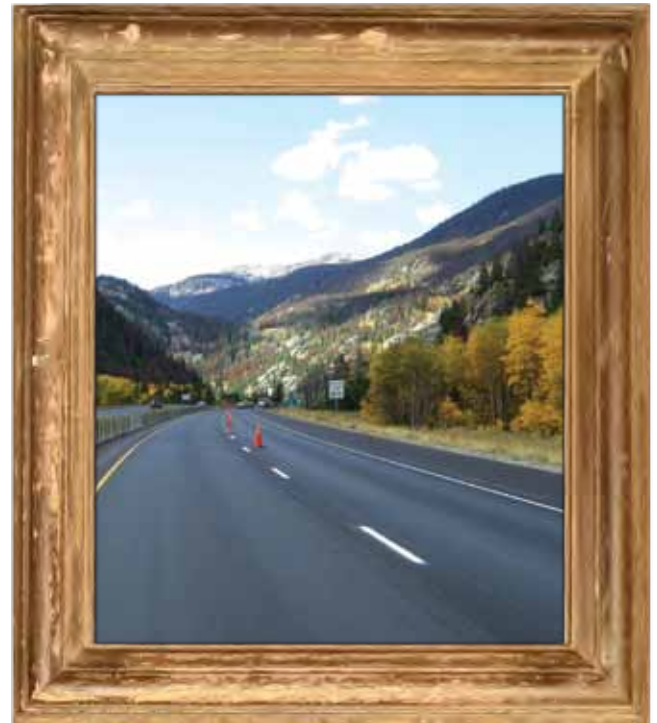
Resurfacing on I-70 between Vail Pass and Silverthorne
