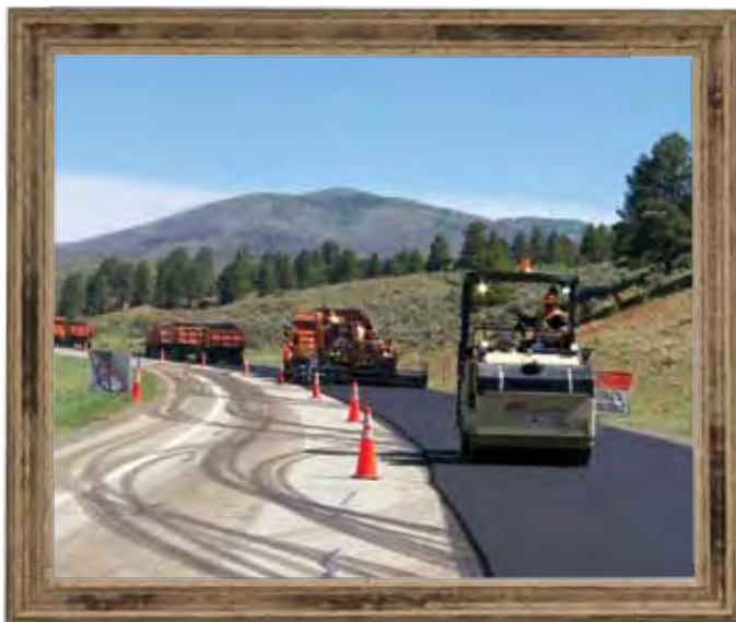
Maintenance resurfacing on US 160 La Veta Pass
