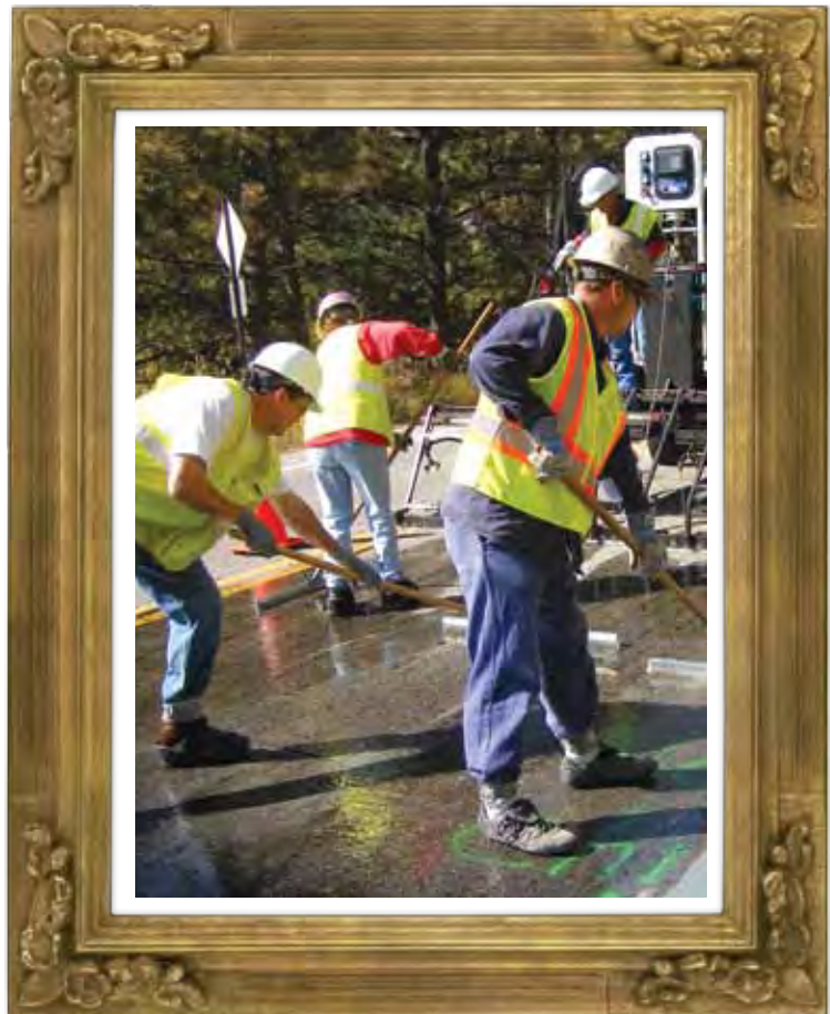
Crews chip seal US 36 near Estes Park
