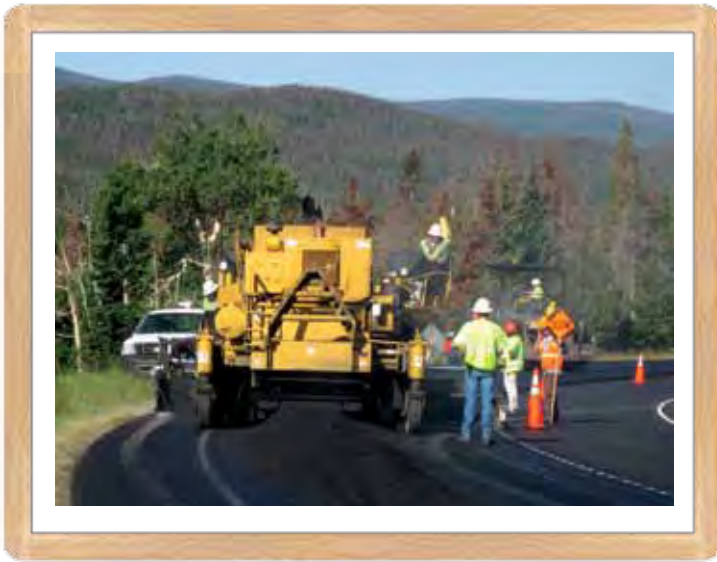
Resurfacing on SH 14 over Cameron Pass
