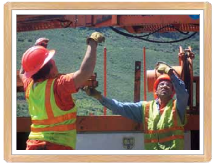
CDOT bridge crews conduct bridge inspection
