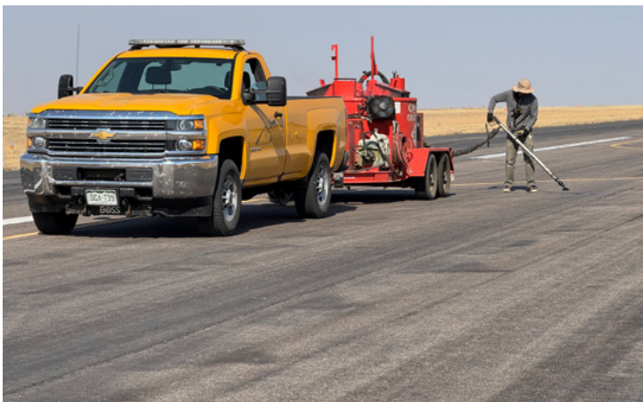
Photo above: Airfield maintenance crews at Burlington-Kit Carson County Airport (ITR) in Burlington, Colorado, apply pavement crack sealer to Runway 15/33. In 2024, ITR received $3,700 in state funding to purchase crack sealing materials. The airport’s crack sealing operations are performed using a machine funded by the Colorado Division of Aeronautics. Photo by Daniel Melia - ITR.
