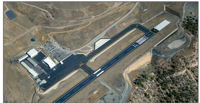
Telluride Regional Airport (TEX) was awarded a $250,000 Discretionary Aviation Grant for airfield pavement maintenance.
