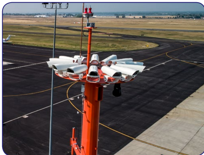
A closer look at the center 360-degree camera array for the Colorado Remote Tower Project at the Northern Colorado Regional Airport (FNL). Photo by Shahn Sederberg
