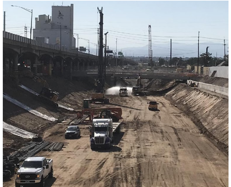
A water truck at work in the lowered section.
