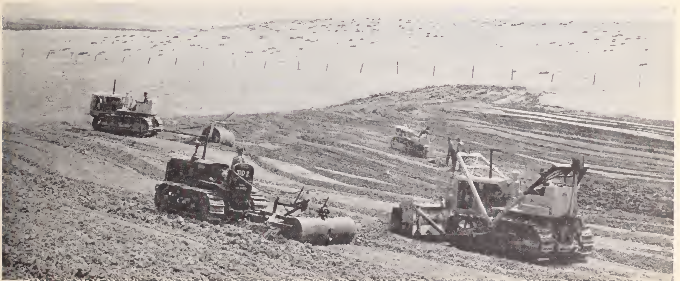
Tractor crew at work on Soil Conservation Service Project—Camp SCS-3-C, Hugo
