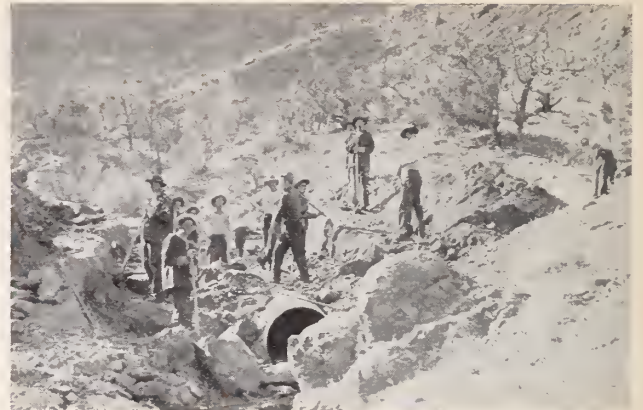
Setting culvert in road Camp NP-9-C, Grand Junction
