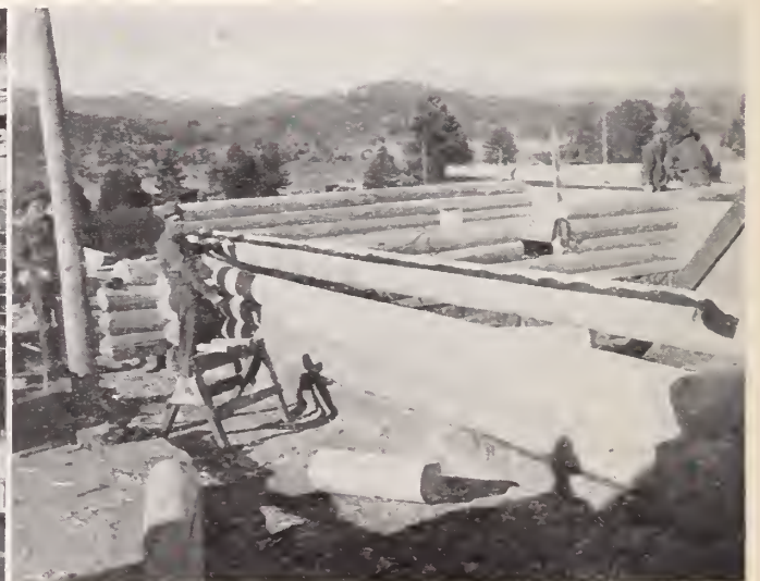
Log work at Lake George Ranger Station Camp F-64-C, Woodland Park
