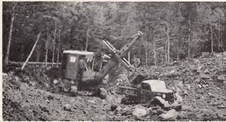
Power Shovel Operation Loading truck—Camp NP-4-C, Estes Park
