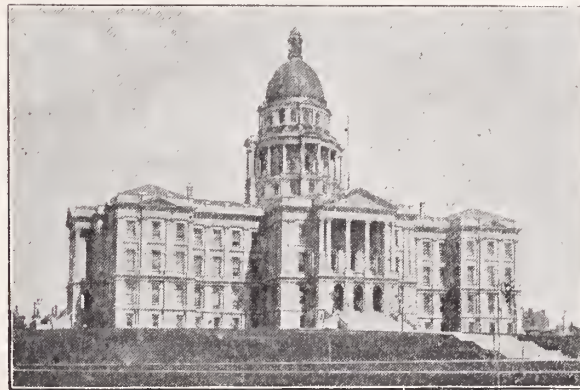
Colorado State Capitol Denver, Colorado
