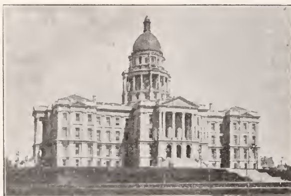
Colorado State Capitol Denver, Colorado
