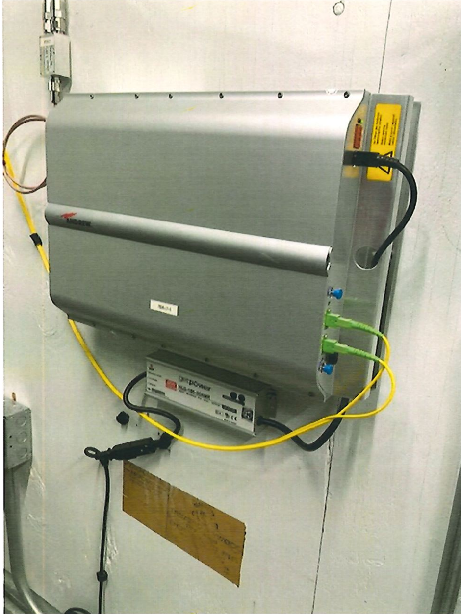
Distributive Antenna System (DAS) Repeater
