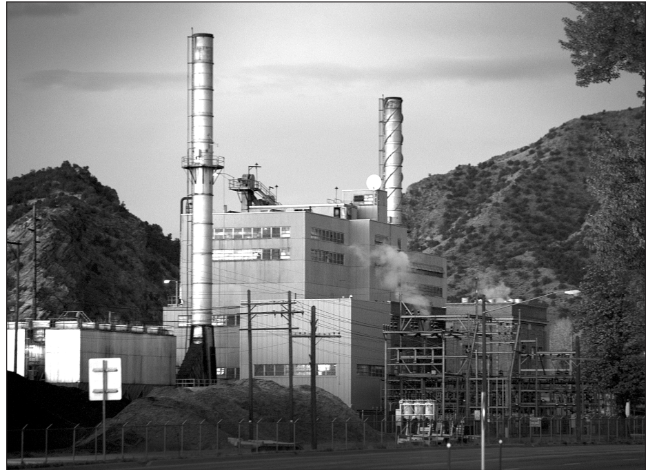
The W.N. Clark electric generating station in Canon City, owned by Black Hills, will be retired under an emissions reduction plan approved by the Public Utilities Commission. (Photo courtesy of Black Hills.)
