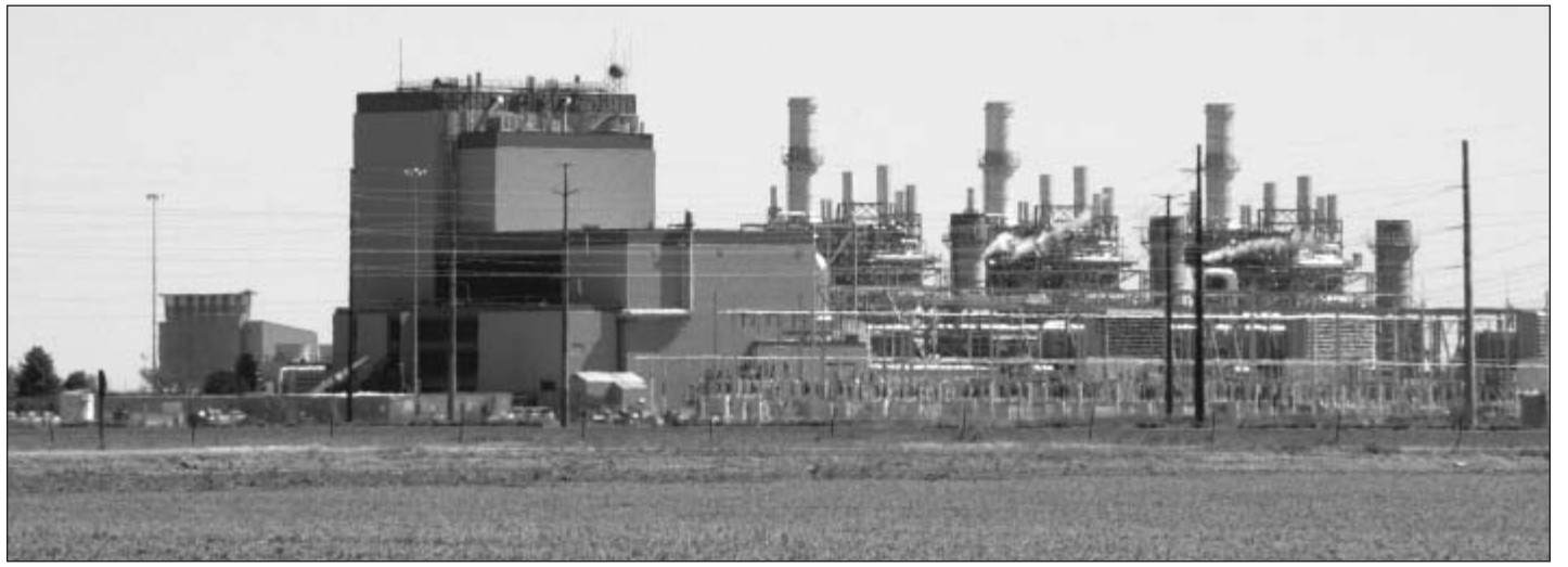
The former Fort St. Vrain nuclear plant near Louisville was converted to a natural gas generating station in the late 1990s. (Photo courtesy of Xcel)
