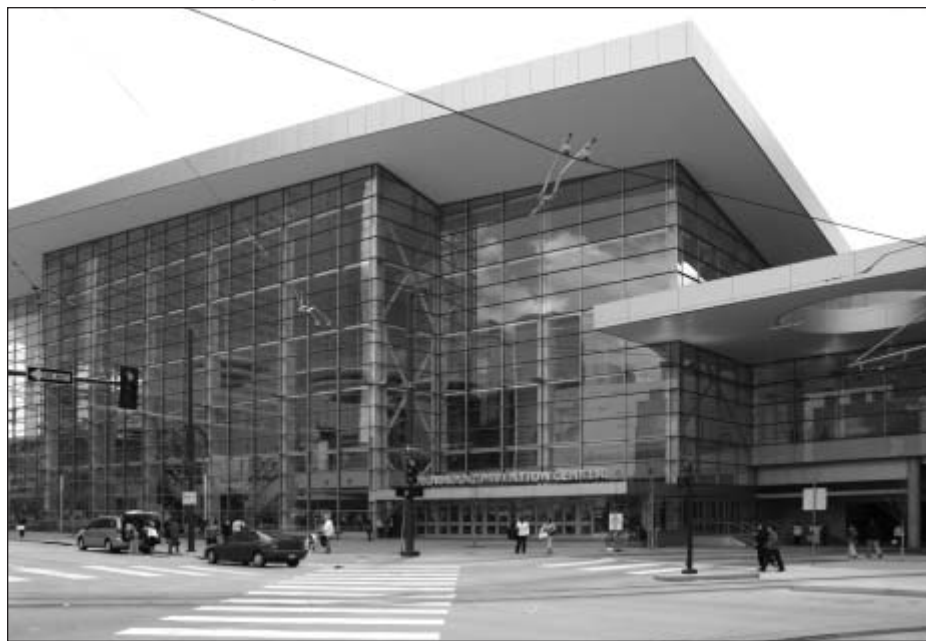
Qwest has filed to recover the costs of moving its facilities to make way for the new Colorado Convention Center, as well as the widening of I-25.
