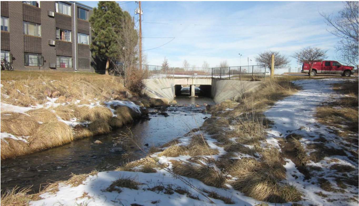
Montview Boulevard box culvert to be replaced on Westerly Creek
