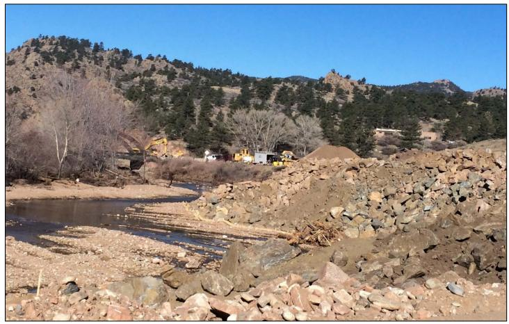
Rock debris from construction blasting along Highway 36 in March 2014 north of Lyons was donated to a number of municipalities to use for their stream bank stabilization projects under the Emergency Watershed Protection grant program.
