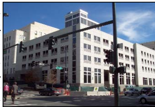
The new parking structure is near completion.
