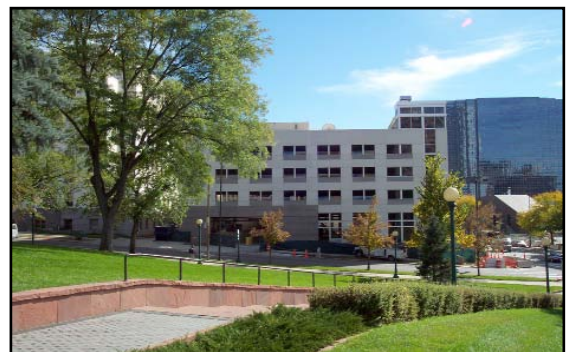
The new structure, looking South, from the Capitol Grounds.
