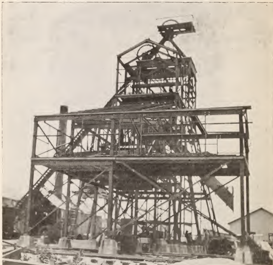
MINE 22—WESTERN COAL AND MINING COMPANY—In Construction One of the Eleven Tipples Built By Us in 1926
