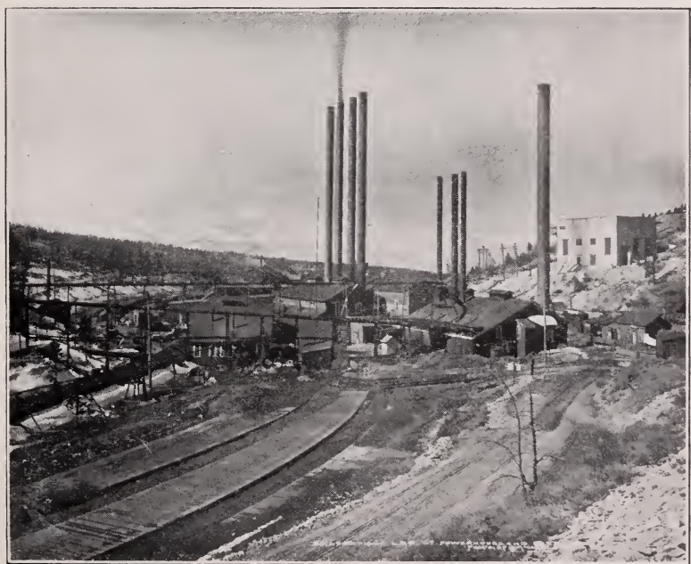
Emergency Steam Plant of The Colorado Power Co. at Leadville; 100,000-Volt Transformer Station in Background.
