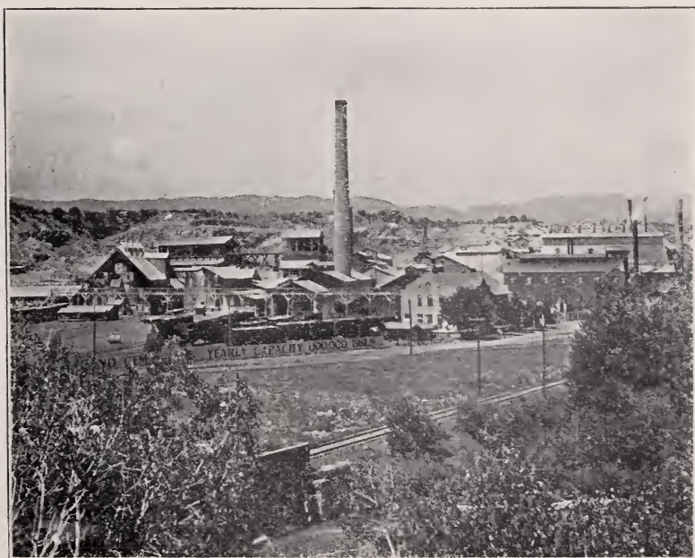
Colorado Portland Cement Co.'s Plant at Portland, Colo. (Nearer View of Plant.)
