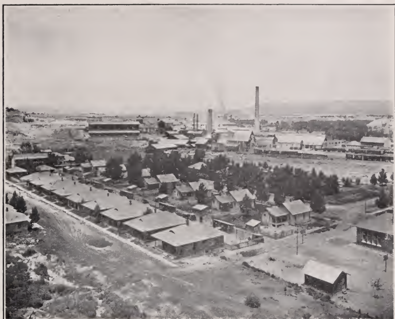
Colorado Portland Cement Co.'s Plant, at Portland, Colo. (Showing Workmen's Homes.)
