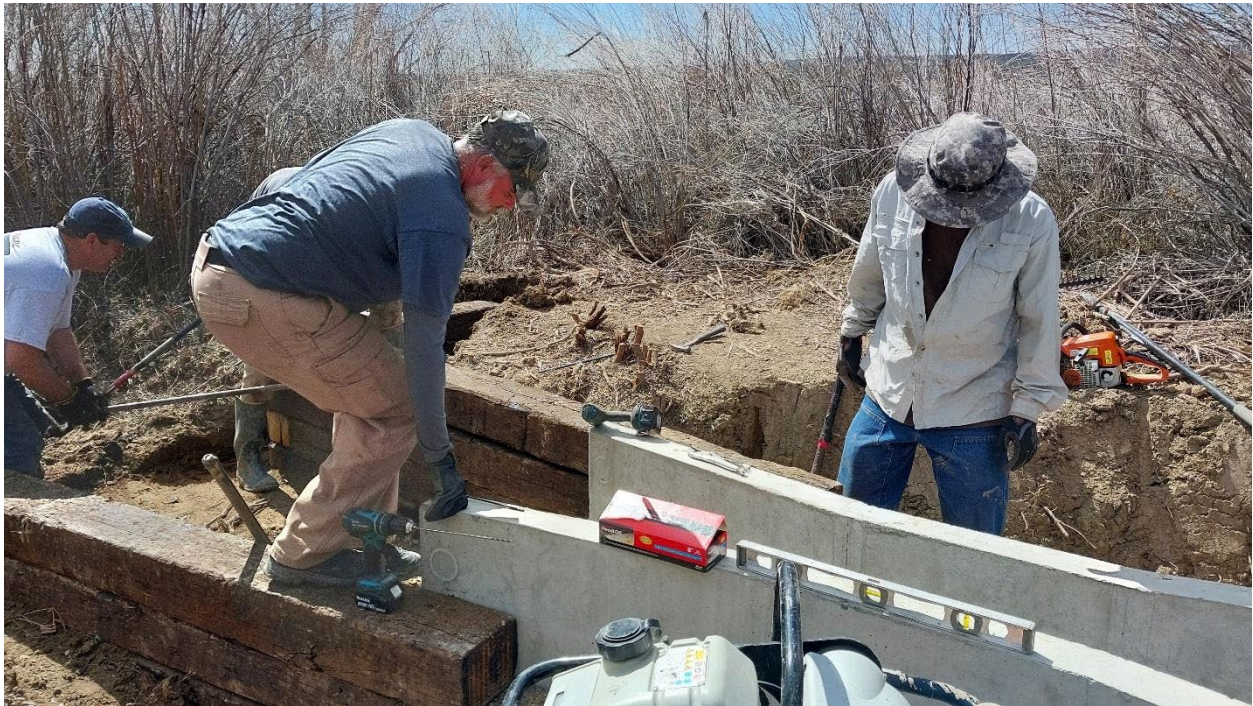
Figure 3: DWR staff installing new Pioneer Ditch Gauge.
