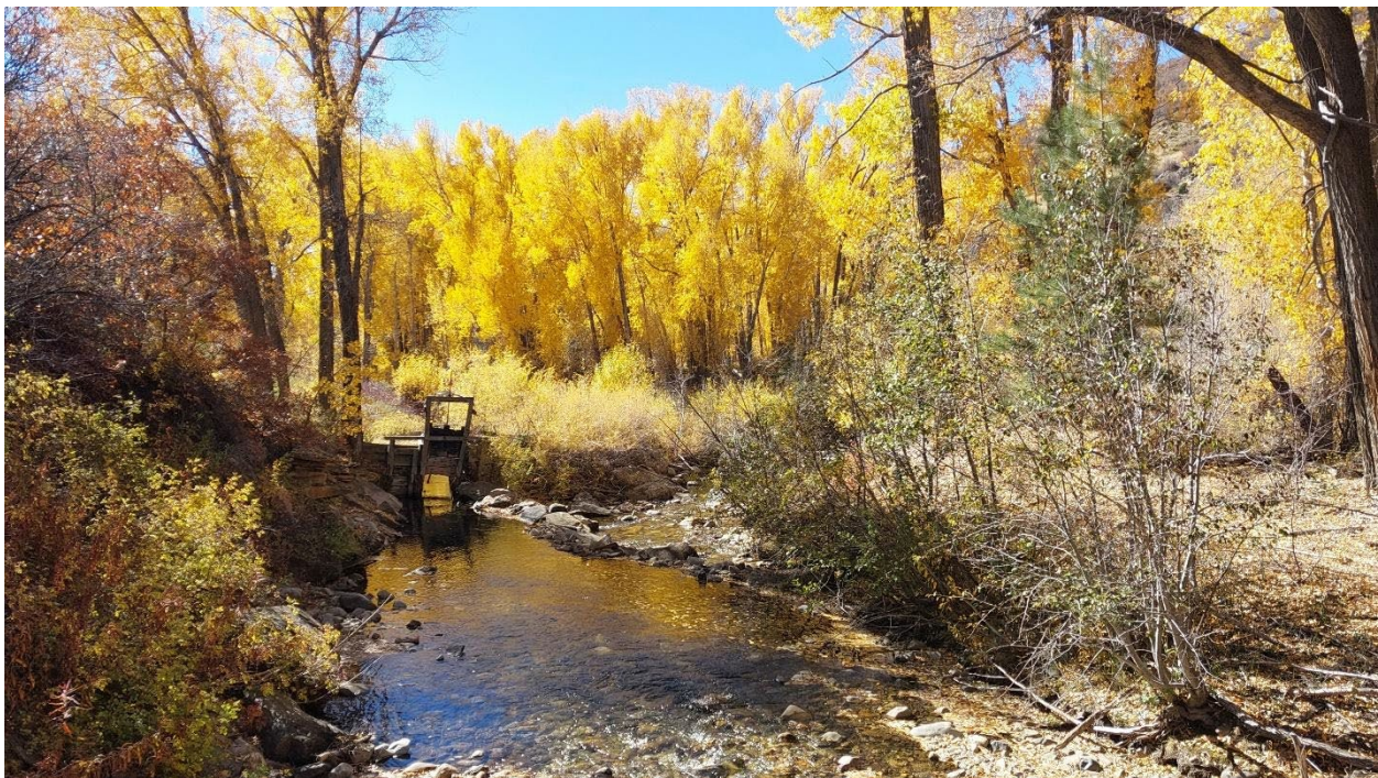
Figure 5: Headgate at La Plata Irrigating Ditch, the Number 1 Priority on the La Plata River.
