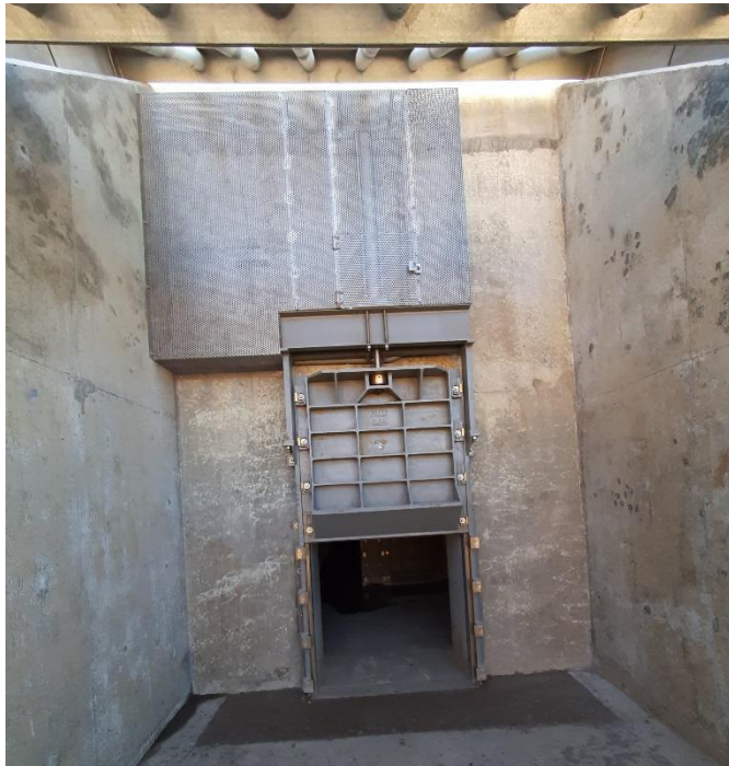
Figure 4: Guard gate leading into outlet structure. Grating above.
