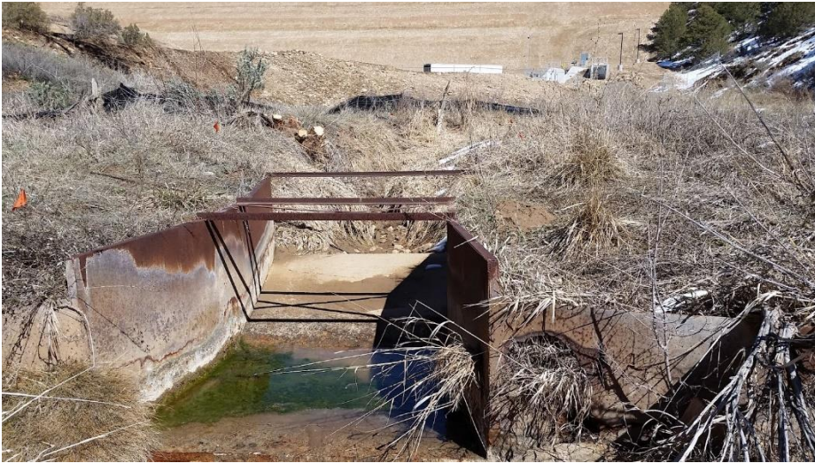
Figure 5- Long Hollow flume prior to replacement
