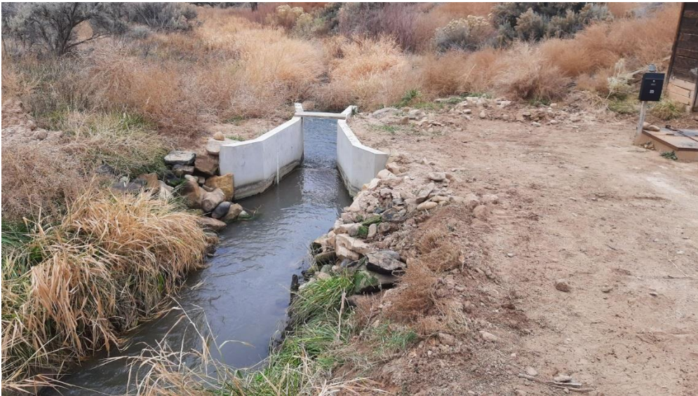
Figure 6 - Long Hollow flume after replacement
