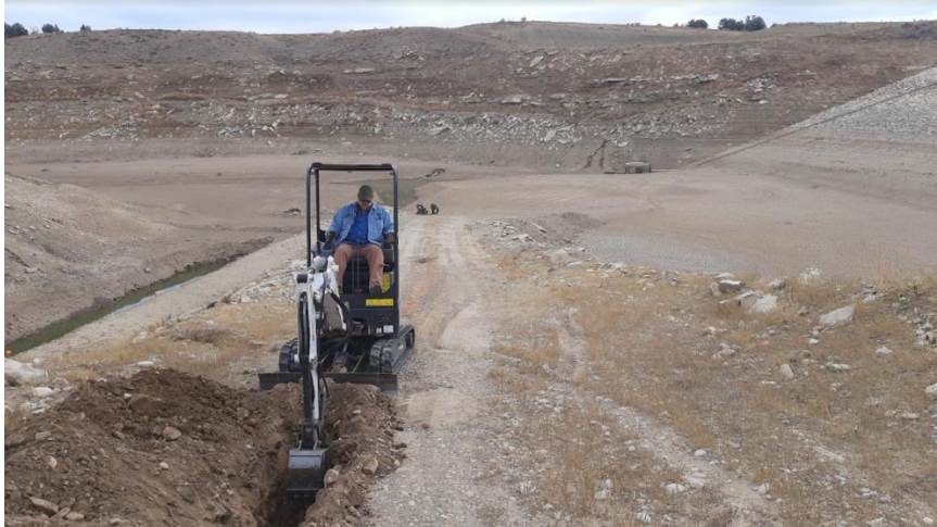
Figure 4 - Installation of conduit in Long Hollow Reservoir
