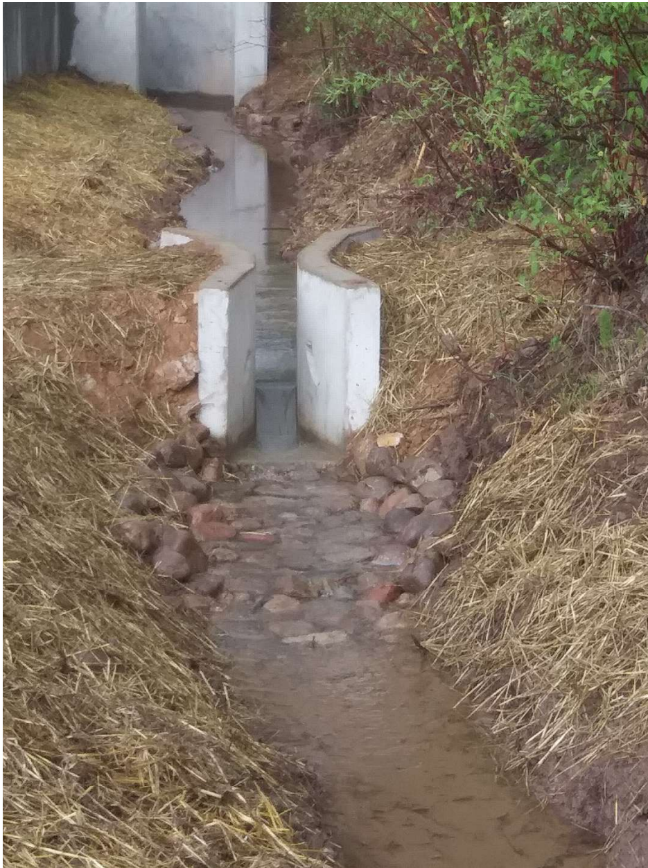
Figure 7: City of Durango Bypass Flume
