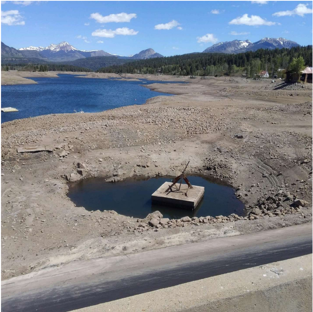
Figure 4: Cascade (Electra) Reservoir drained for repairs
