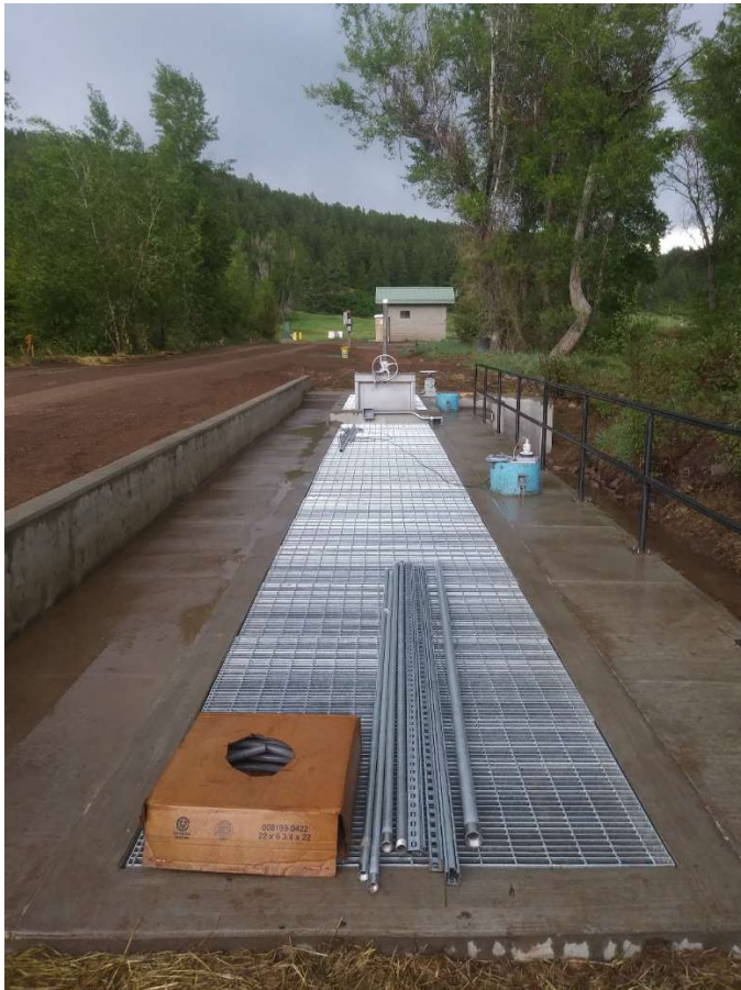
Figure 6: City of Durango Flume on the Florida River
