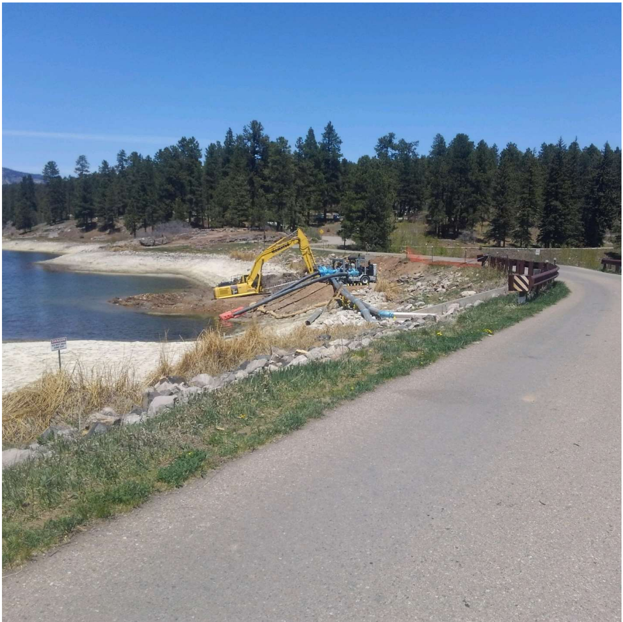
Figure 5: Draining of Haviland Lake to repair outlet structure
