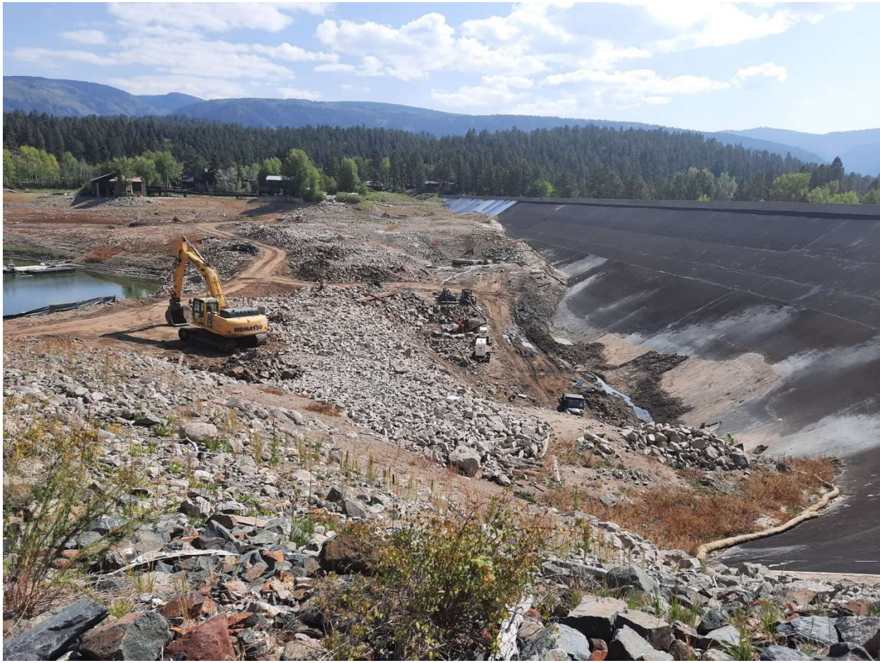
Figure 3: Upstream face of dam at Cascade (Electra) Reservoir
