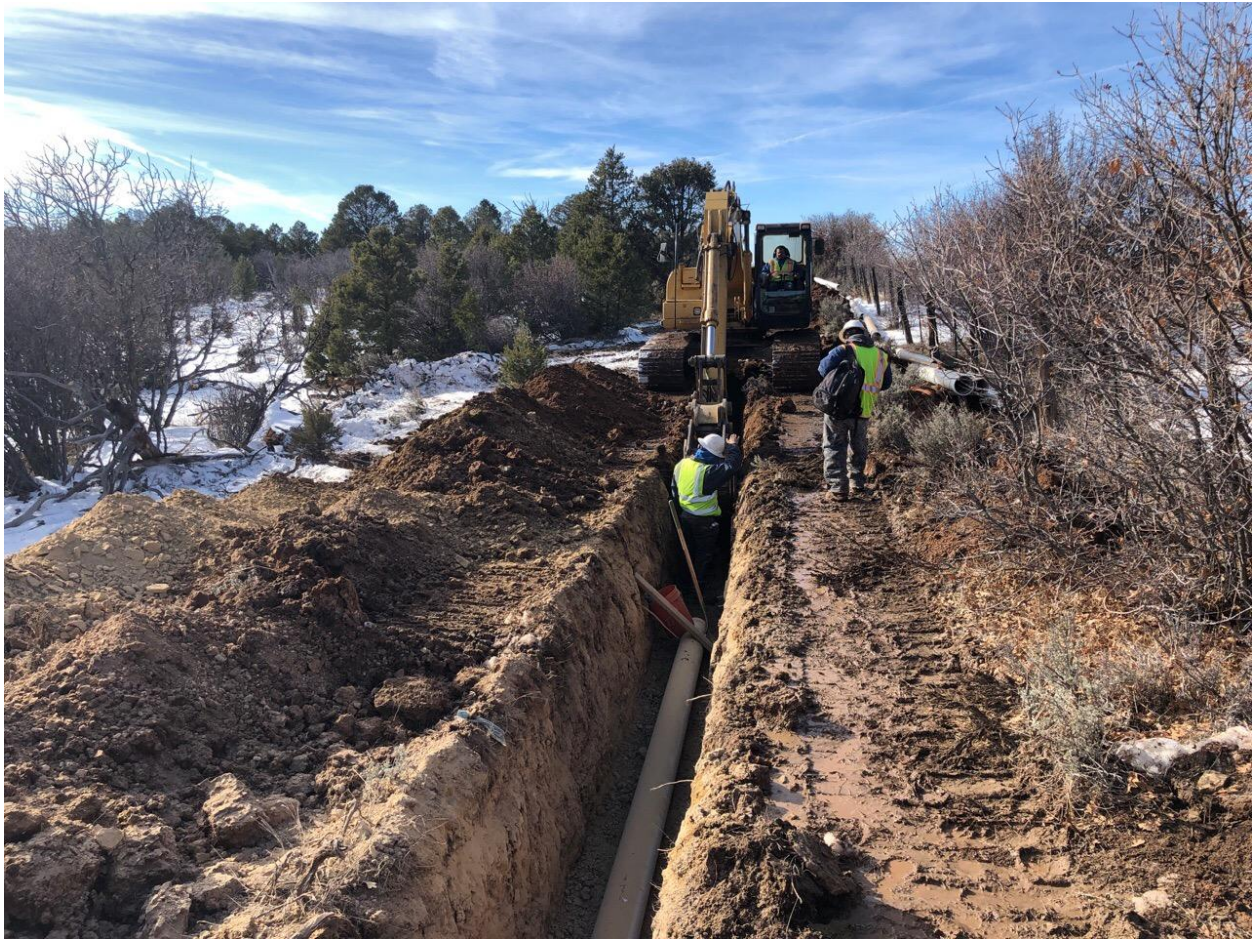
Figure 5: Lake Nighthorse to Lake Durango Pipeline Construction
