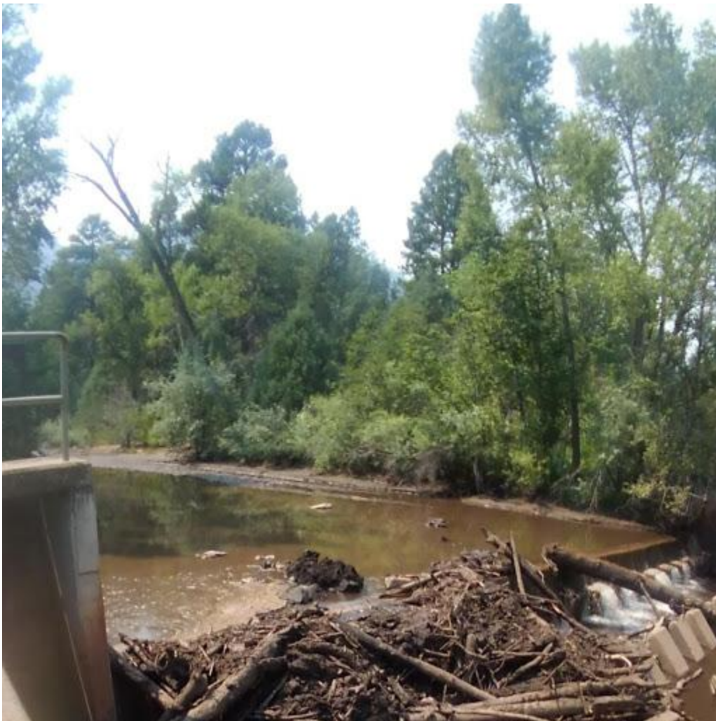
Figure 1: Fire debris collecting on the Hermosa Company Ditch headgate, downstream from 416 Fire
